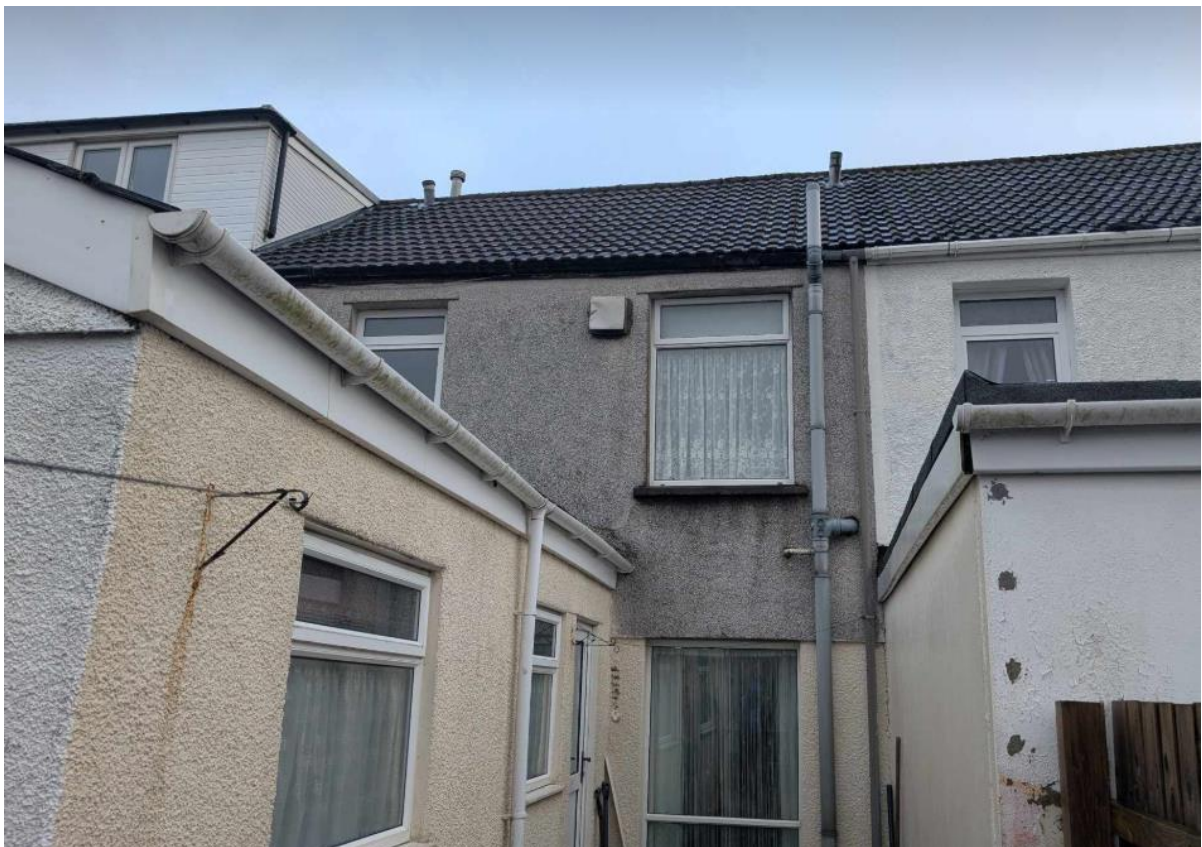
Plate 8- photograph of rear roof
