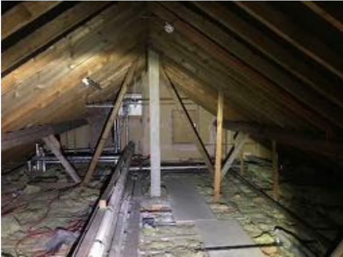
View of internal attic space
