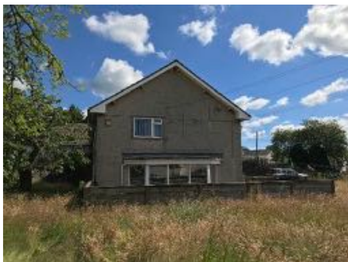
South gable end of building
