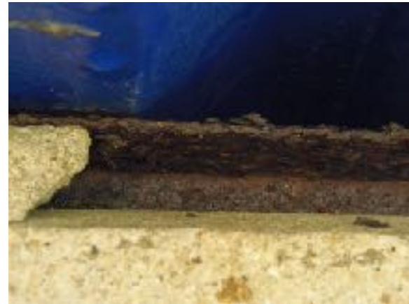
B1 - roofing sheet sitting on metal girder at rear
