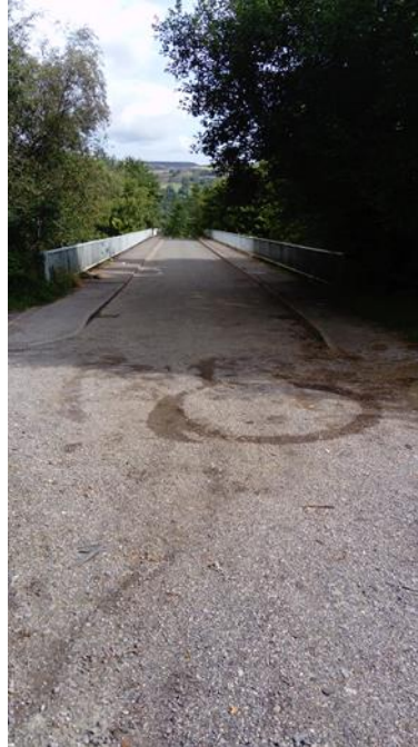
Plate 3.2: Bridge over A470
