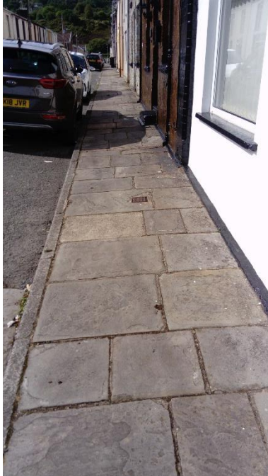
Plate 3.6: Footways along Cardiff Street
