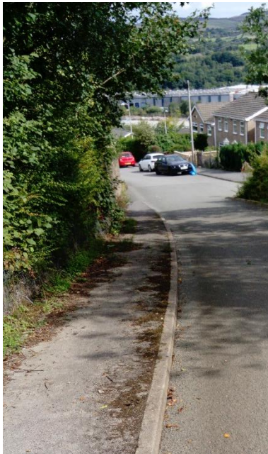
Plate 3.3: Footway along western side of Graig Road
