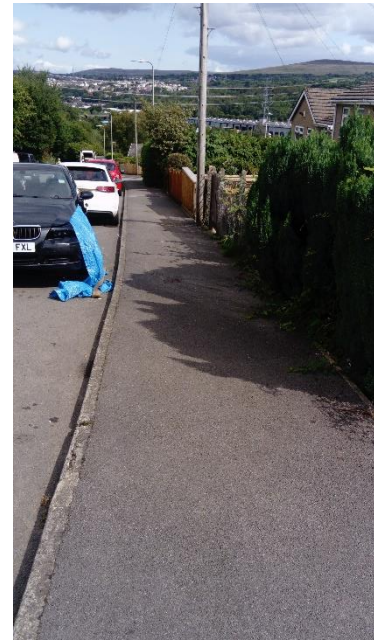
Plate 3.4: Footway along eastern side of Graig Road
