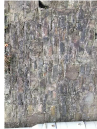
New Stone Wall to Match existing
