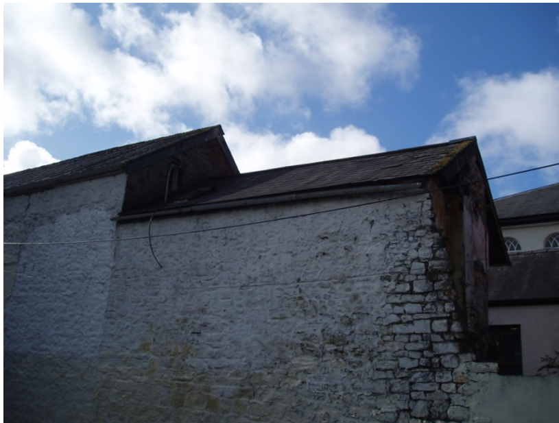
The side elevation of the building in Old Mill Lane
