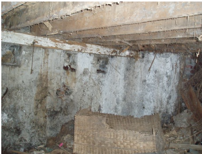
Internal views, loft space top (asbestos sheeted section), typical condition of rooms apart from the former shop, below.
