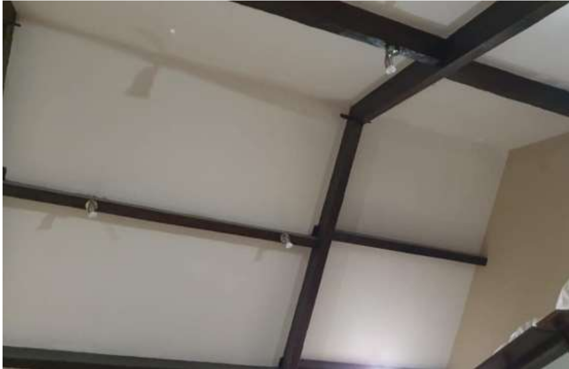
Plate 10- Photograph of vaulted ceiling
