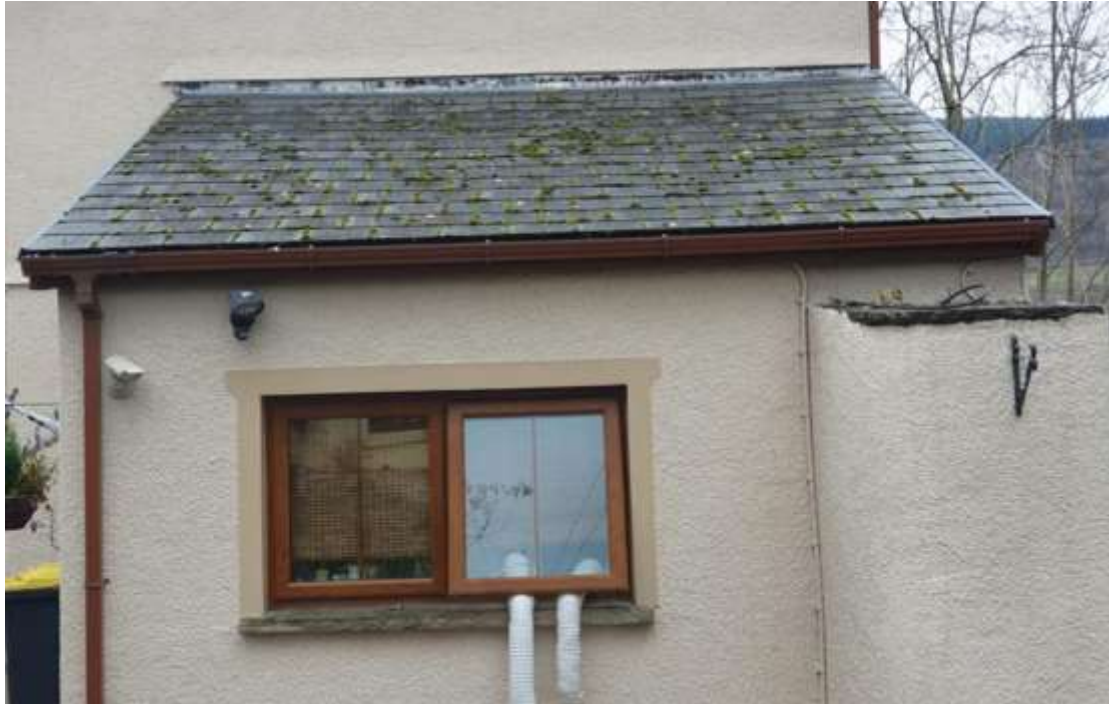
Plate 9- photograph of relatively well sealed porch
