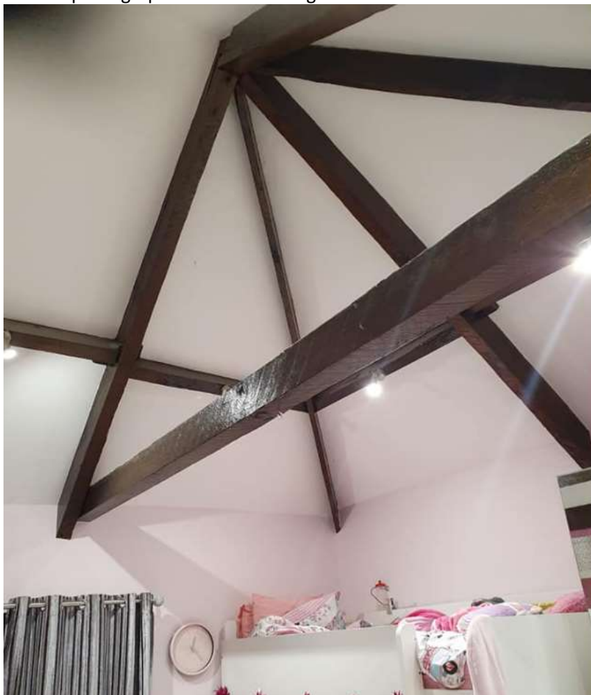
Plate 9- photograph of vaulted ceiling
