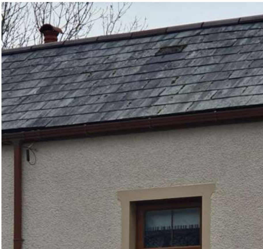
Plate 8- photograph of relatively well sealed roof with small number of slipped slates
