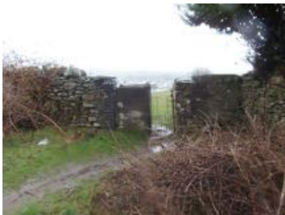
Access to field in south east corner
