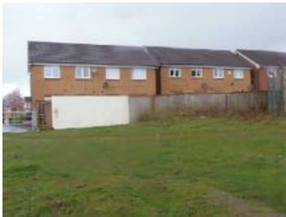
Section of western boundary of breeze block
