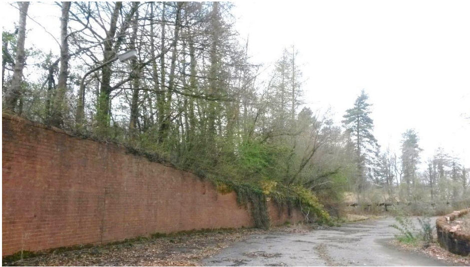
Plate 3-3: Retaining wall on the eastern site boundary treeline
