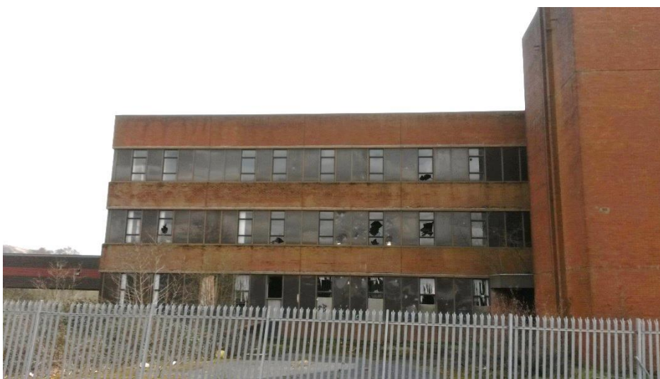
Plate 3-5: Former office building, northern elevation
