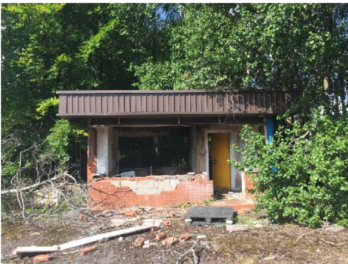
Remaining small building
