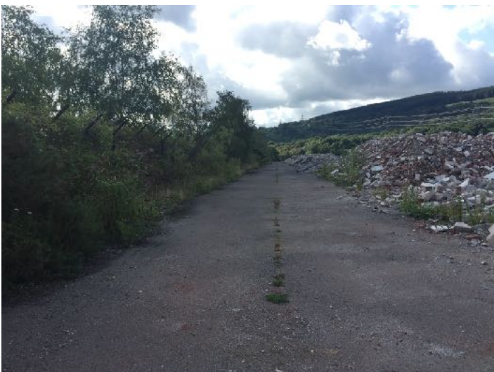
Tarmac road along north east looking south
