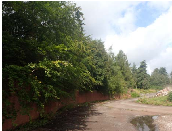
Tree ID#G2 – Retaining wall area
