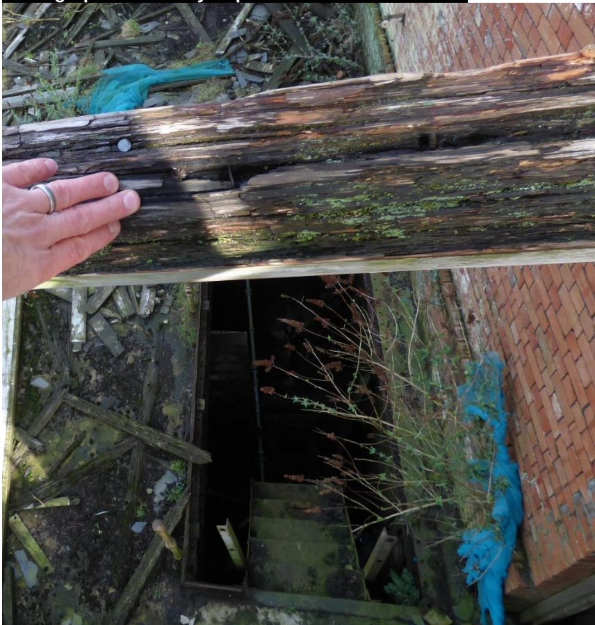
Photograph 22 ~ Decay to purlin and stair well below
