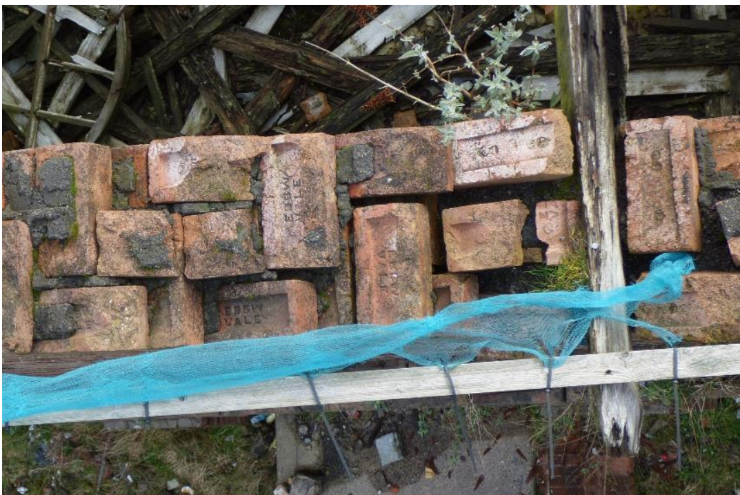
Photograph 15 ~ View from above gable wall and purlin connection
