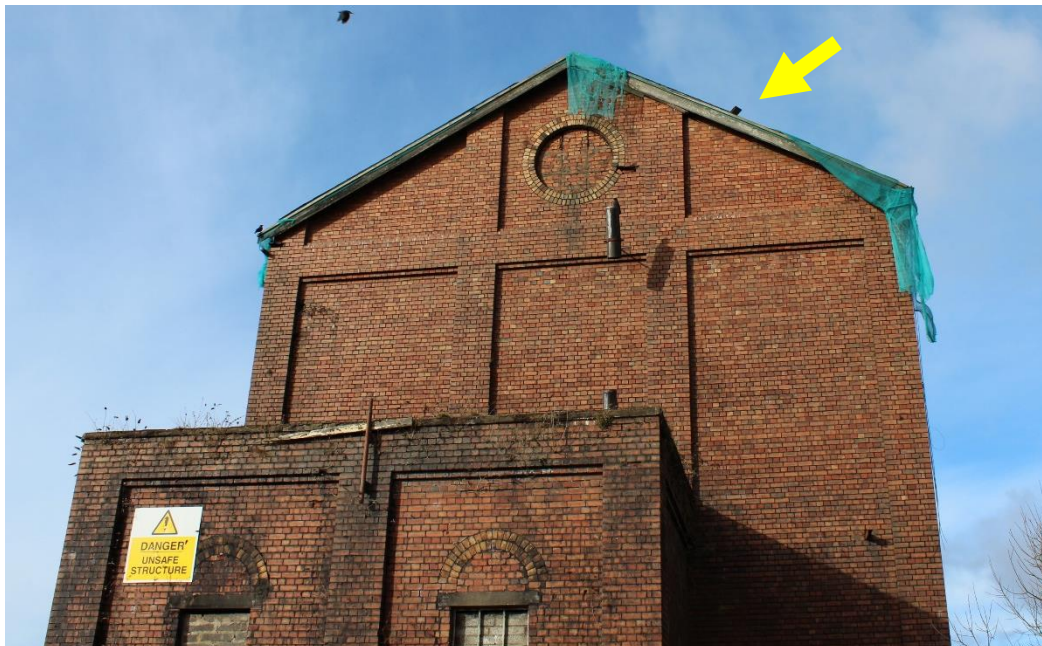
Photograph 5 ~ End east elevation overhanging slate arrowed
