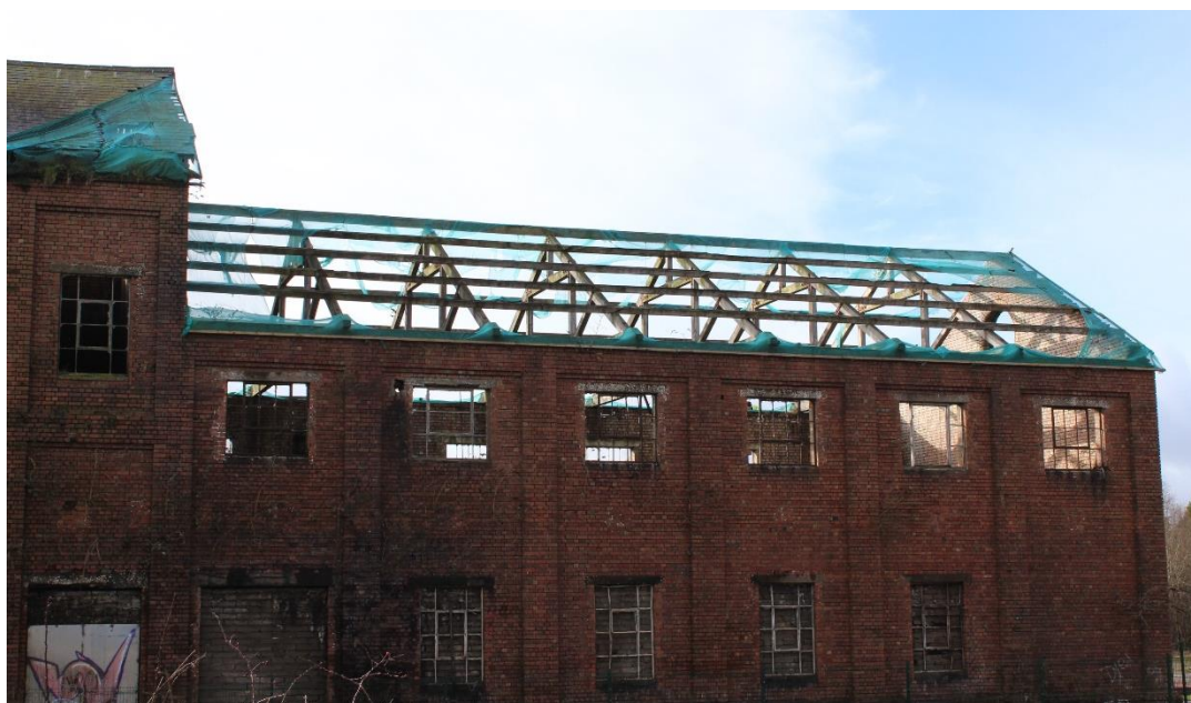
Photograph 11 ~ Rear north elevation
