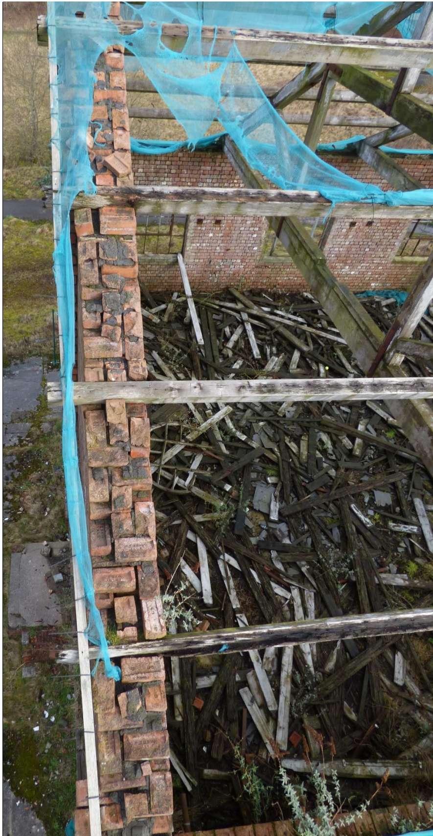
Photograph 16 ~ West gable wall and 4 purlins
