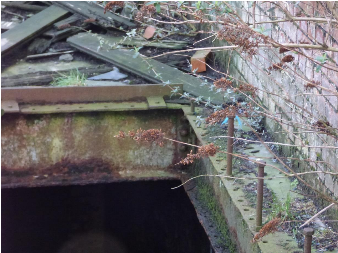
Photograph 22 ~ Decay to purlin and stair well below
