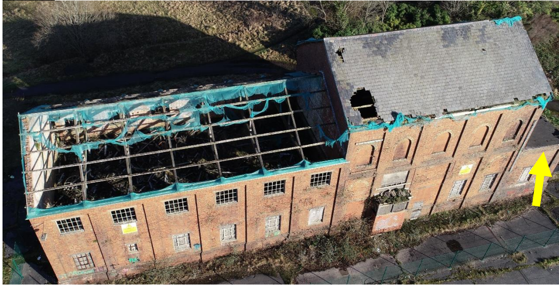
Photograph 12 ~ Roof lower west end to LHS and upper east end to RHS flat roof arrowed
