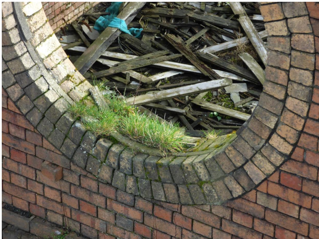
Photograph 17 ~ Circular window in west gable wall
