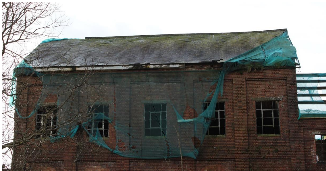
Photograph 10 ~ Rear north elevation
