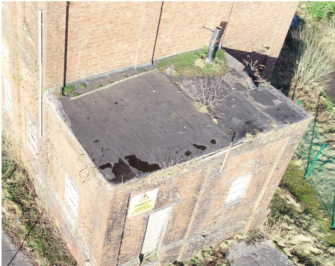
Photograph 18 ~ Flat roof to east end
