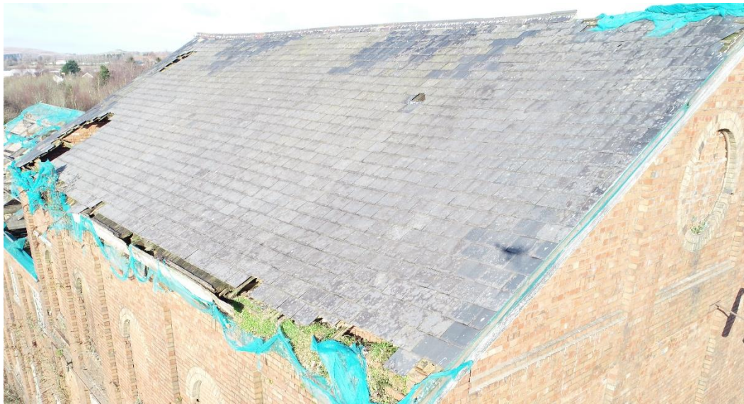
Photograph 19 ~ Front roof pitch to east end
