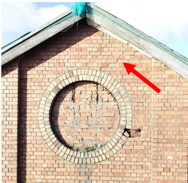
Photograph 24 ~ Crack above blocked in circular window to east end gable
