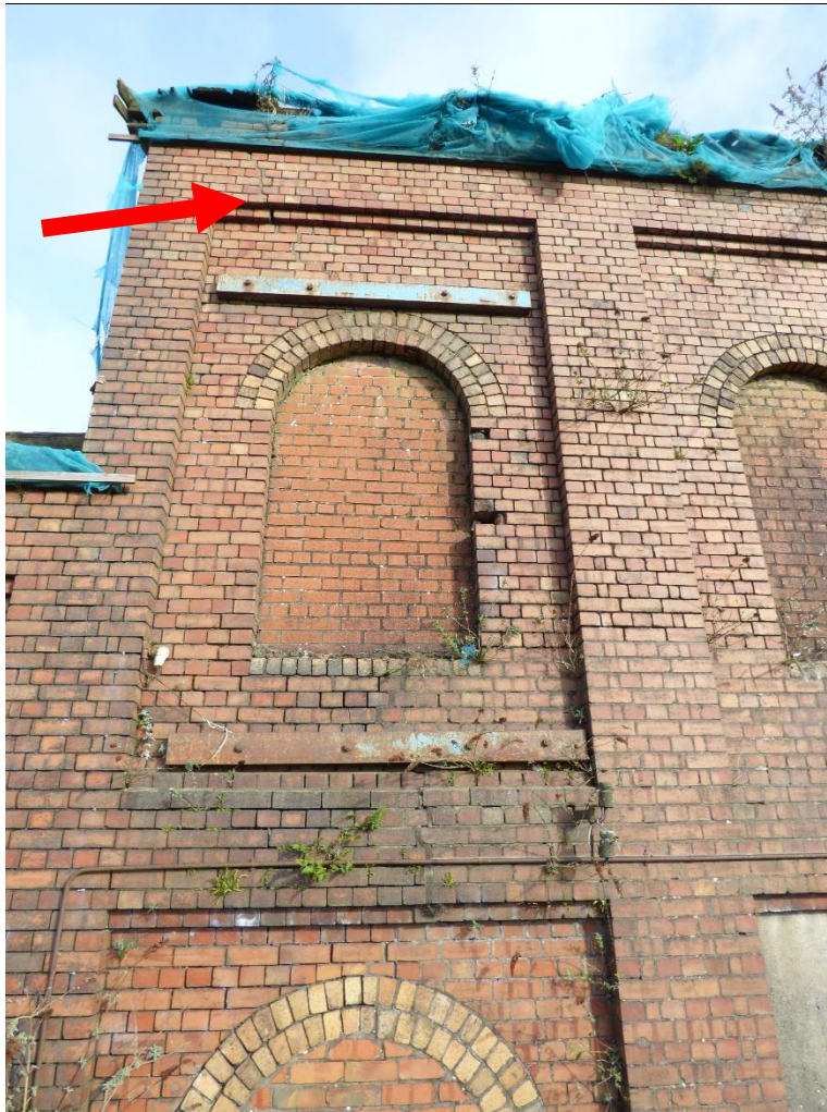
Photograph 24 ~ Crack above blocked in circular window to east end gable
