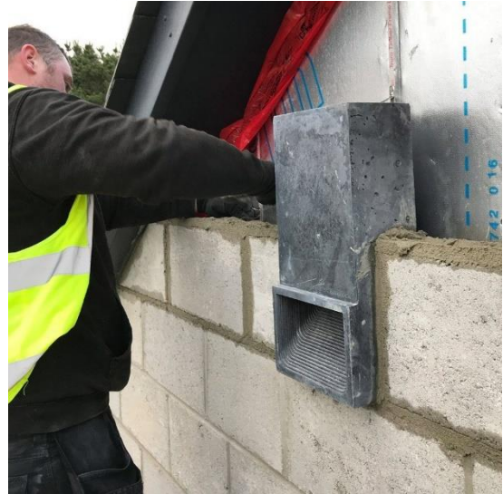
Plate 17: Integrated box in place
