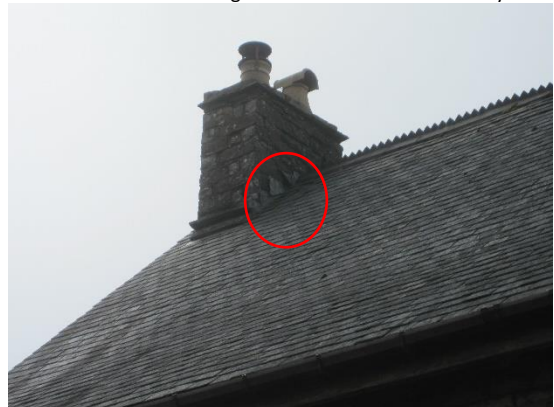
Plate 8: Lifted lead flashing around eastern most chimney
