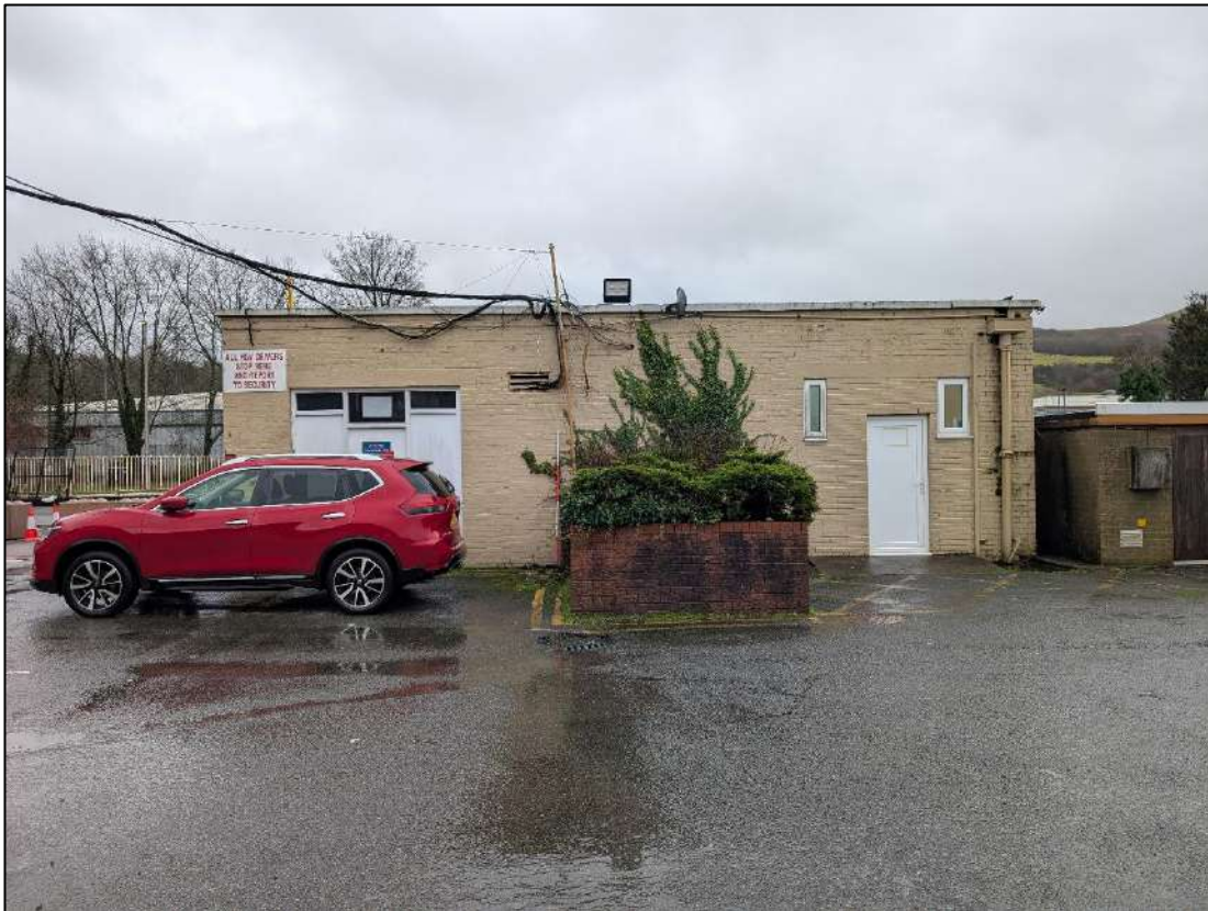
Plate 26. Security hut exterior, view to the east-north-east.
