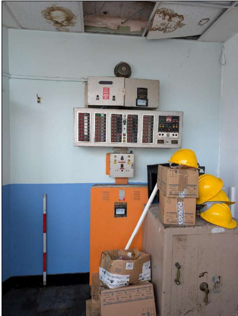
Plate 43. Electrical room, view to the south-east.
