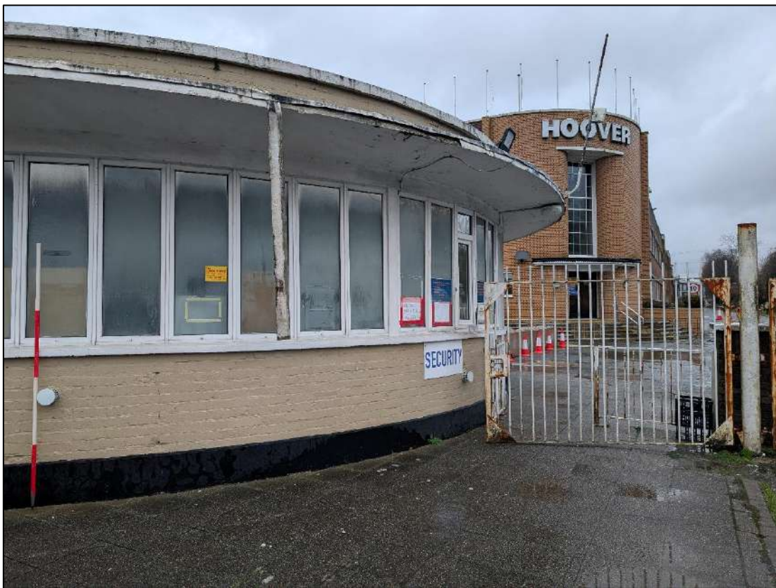
Plate 22. Security hut and main frontage, view to the north-west.
