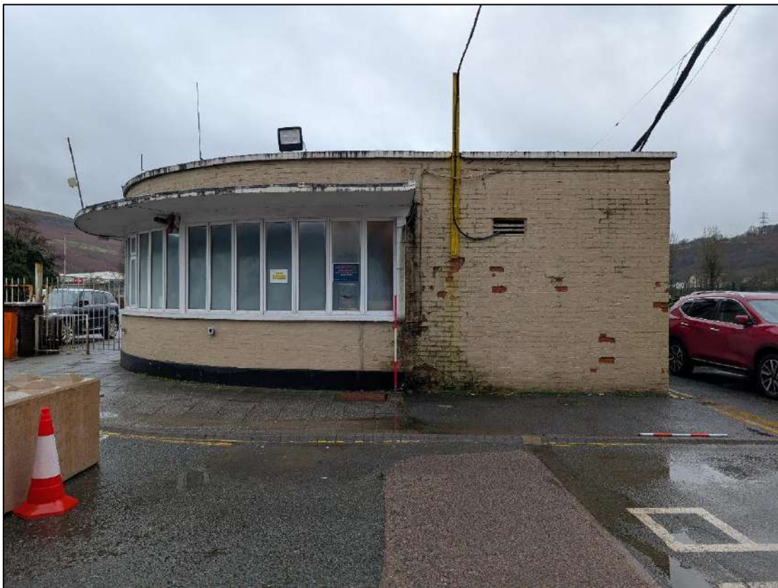
Plate 24. Security hut exterior, view to the south-east.
