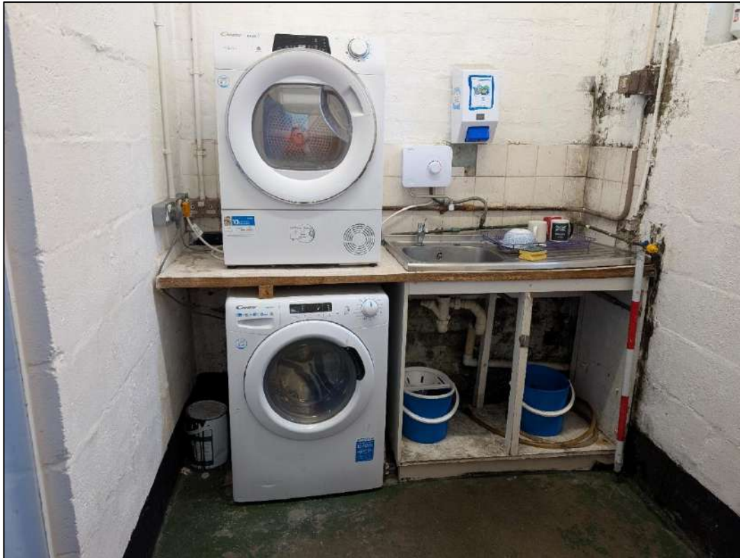
Plate 39. Utility room, view to the south-east.
