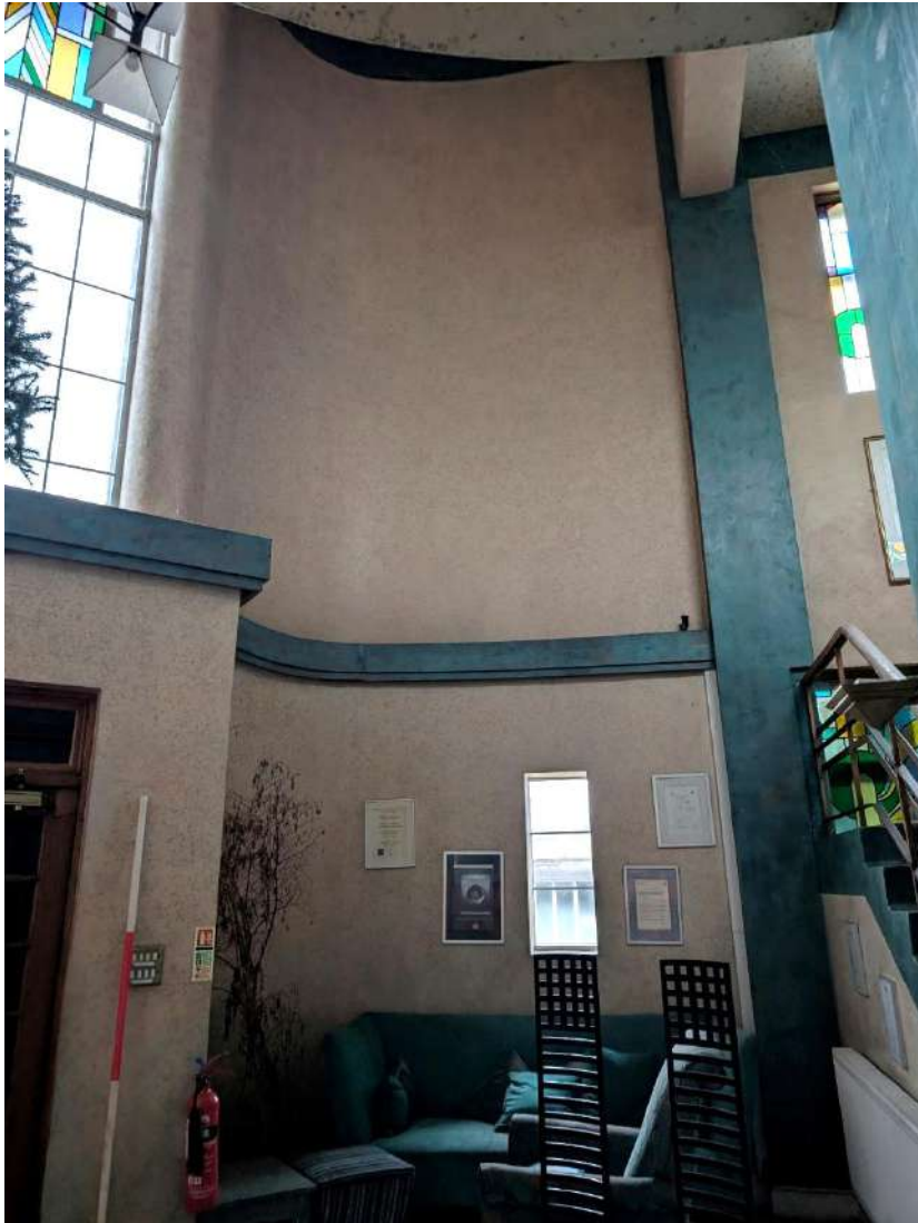
Plate 17. Internal elevation of the frontage, view to the south.
