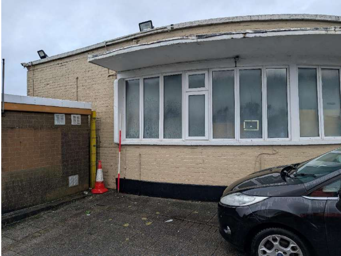
Plate 25. Security hut exterior, view to the north-west.
