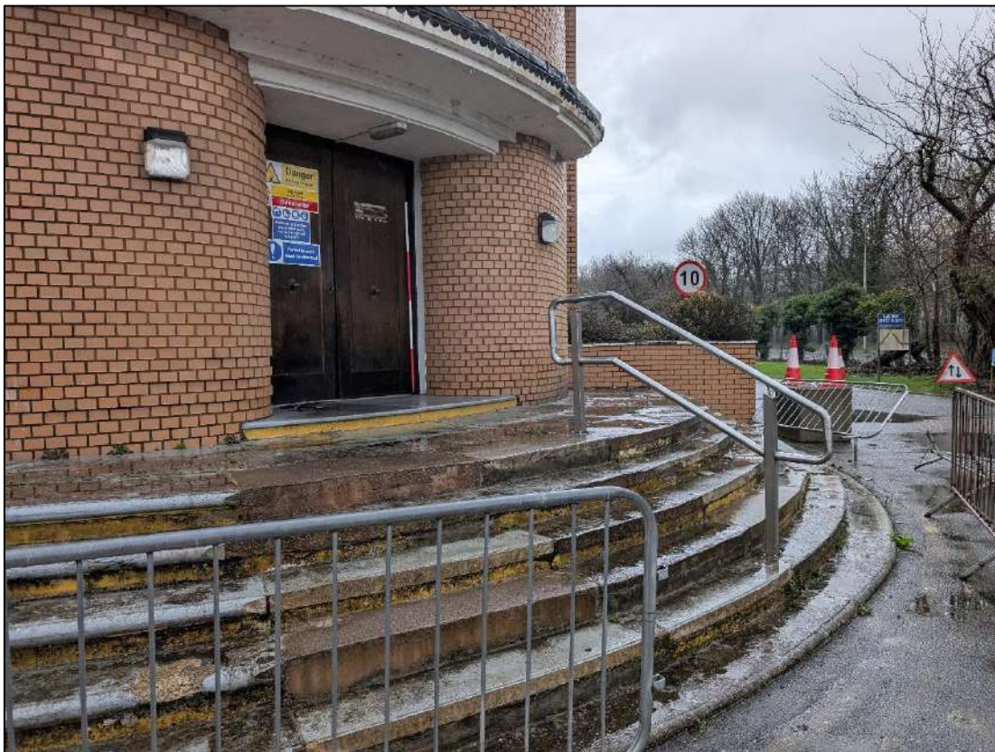
Plate 9. Steps at the main entrance, view to the north.
