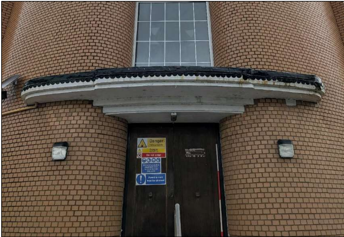
Plate 10. Front door of main entrance, view to the north-west.
