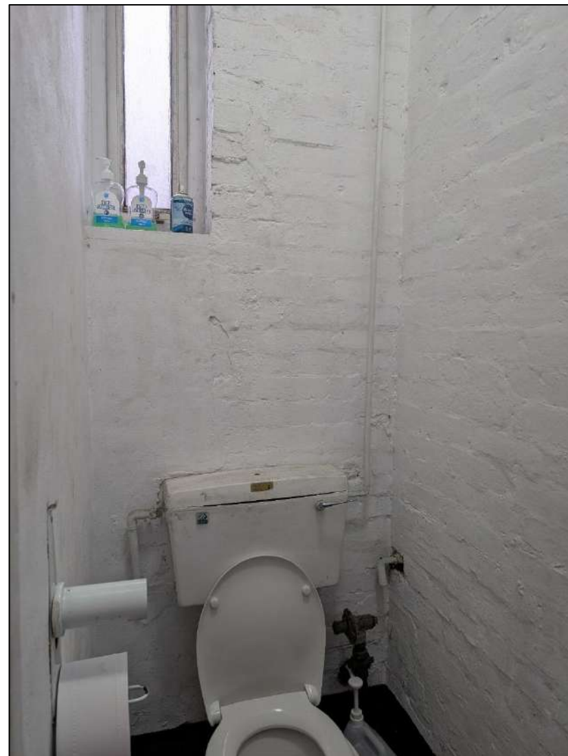
Plate 42. WC, view to the south-west.
