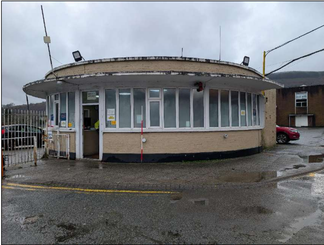
Plate 23. Security hut exterior, view to the south.
