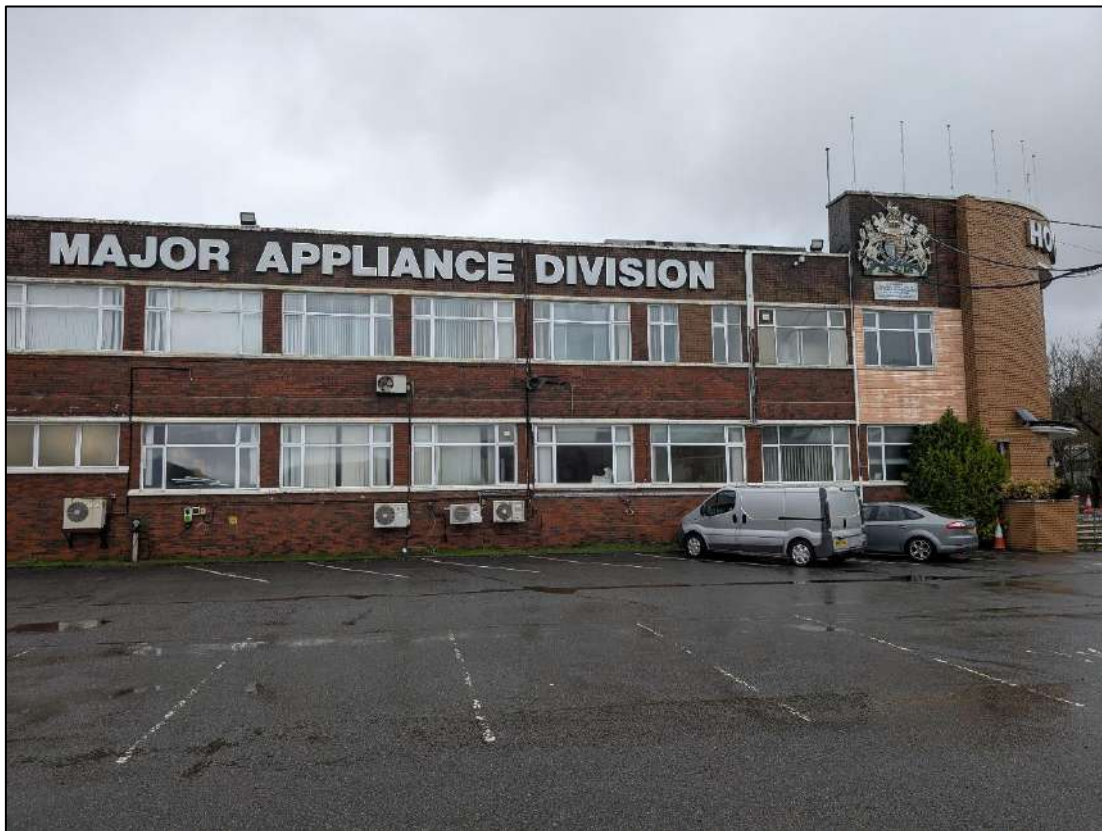
Plate 7. South-east facing elevation of Hoover main building.
