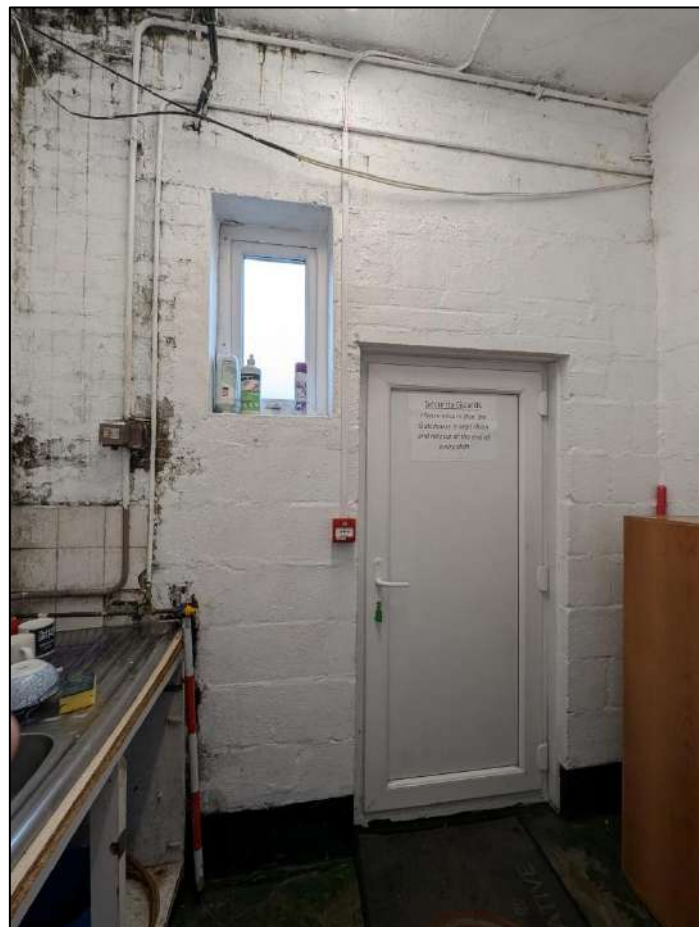
Plate 40. Utility room, view to the south-west.
