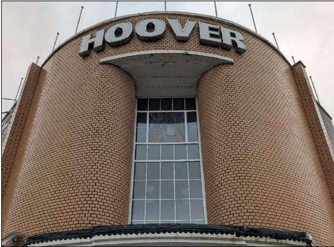
Plate 12. Window within front elevation, view to the north-west.
