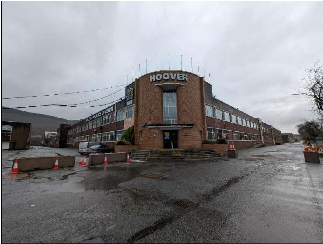
Plate 6. Frontage of Hoover main building, view to the north-west
