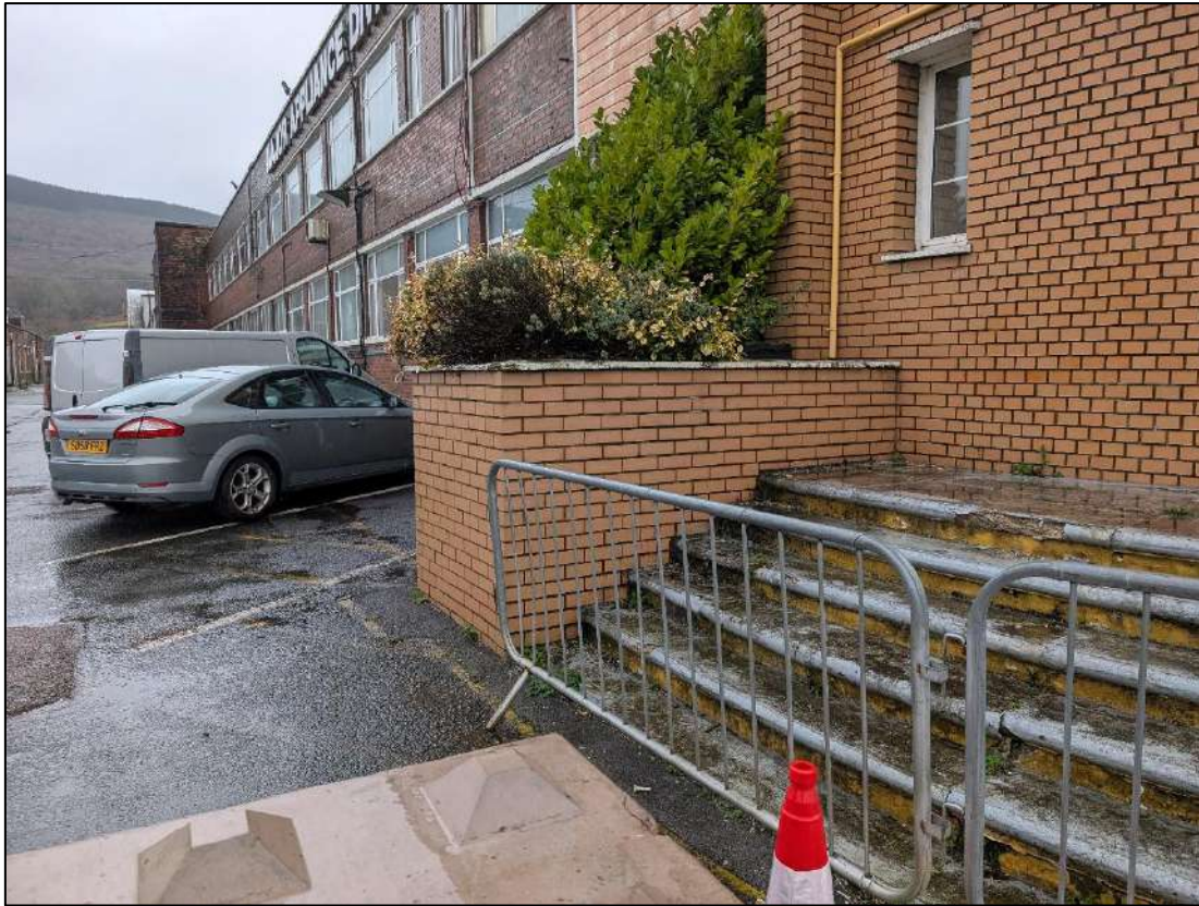
Plate 8. Step end wall and planter, view to the north-west.
