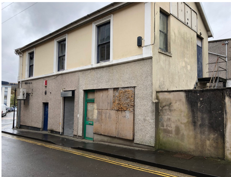
Photograph along Masonic Street to the rear of 32 High Street.
