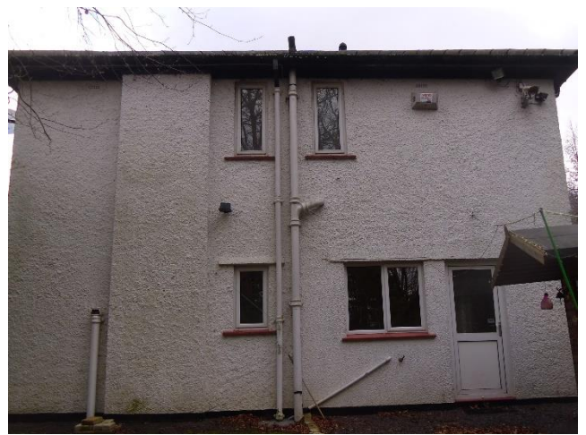
Figure 16: Northern aspect of residential dwelling
