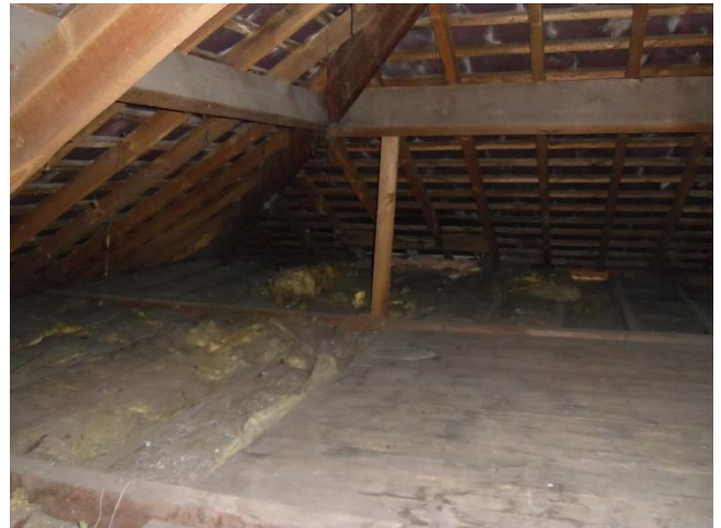
Figure 6: Roof void within residential dwelling
