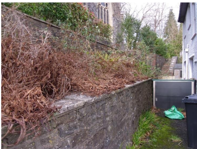
Figure 15: Wall around the western boundary of the site
