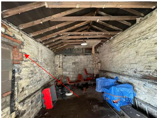
Plate 7: Interior – larger, north-west room, with absence of cavity shown by red arrow
