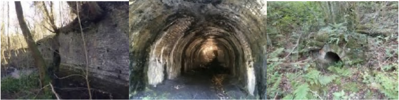
Photos of B12 Cwm Pit retaining wall (left) and recessed tunnel in retaining wall (centre). Photo to the right shows B21 culvert
