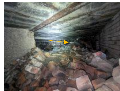
Plate 6 – Interior of building B showing rubble infill and small remaining opening at the adjacent stream.
