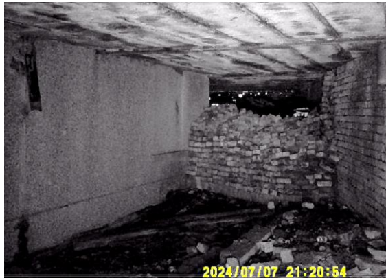
Plate A: Infrared Monitoring (Image quality): showing the interior of Building B
