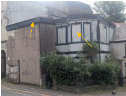
Plate 1 – Western elevation of Building A facing main service road showing flat concrete roof and blocked up window openings.
