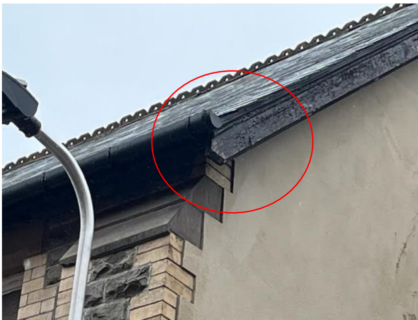
Figure 3: Photograph of approximate emergence point circled red
