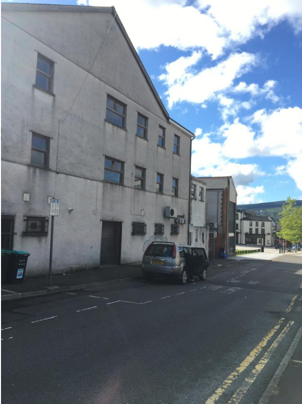
Rear elevation-looking south
