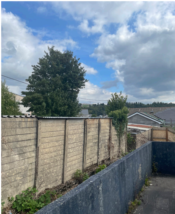
02) Rear of the garages
