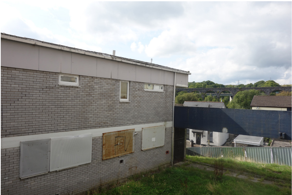
03) View towards the viaduct
