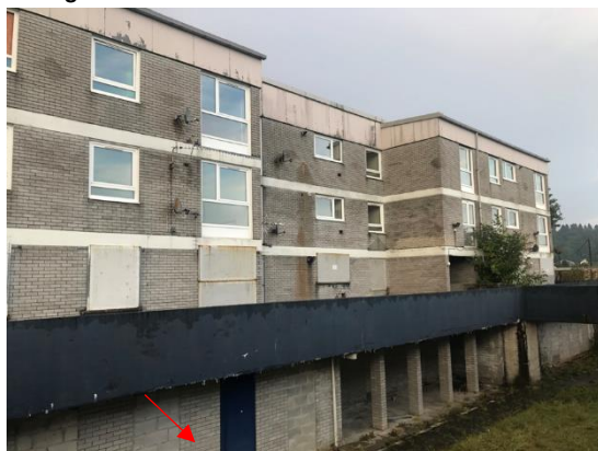
Plate 9: Upper Building, southern elevation, possible emergence location
