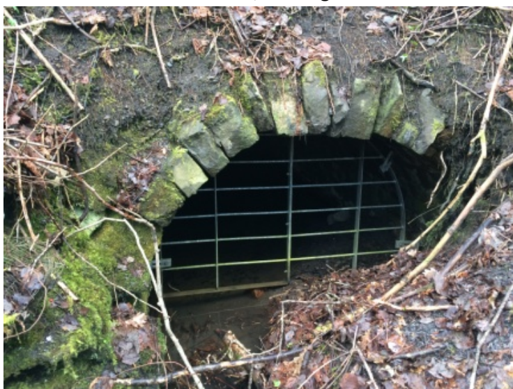
Photo 1: Culvert carrying Nant Cwm Pant Bach to the south of the site and surveyed for bats in 2016 – location marked as D1/A on Figure 3.
