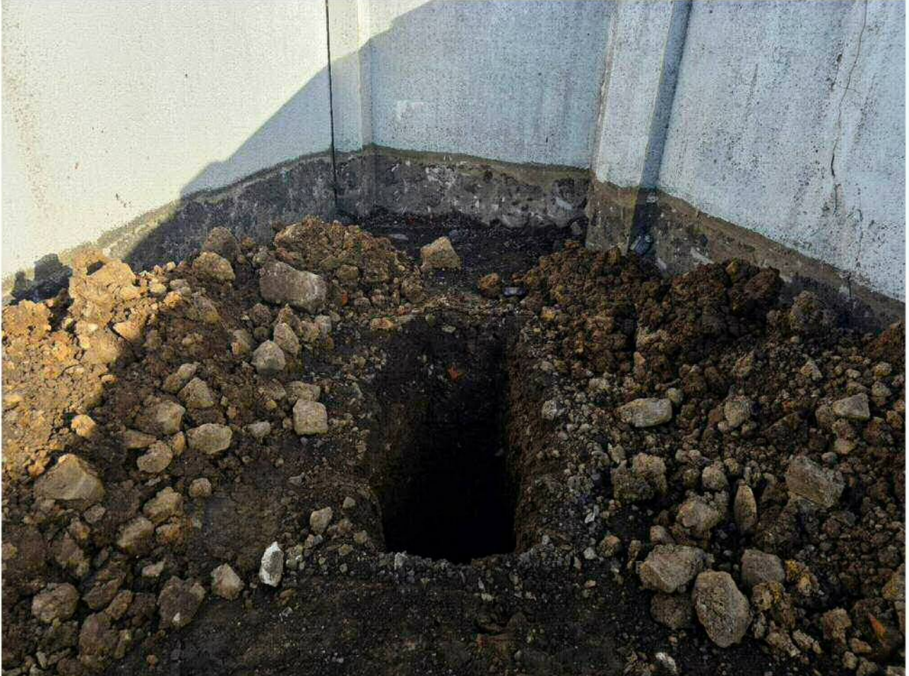
Figure 2 - Test pit 1 during excavation
