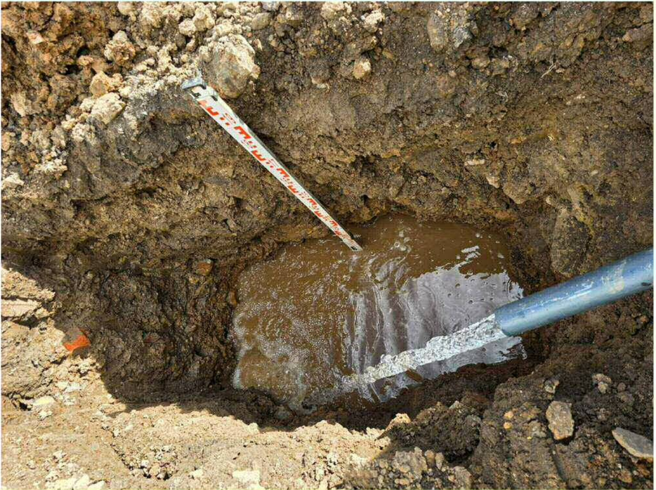
Figure 4 – Test pit 1 during filling
