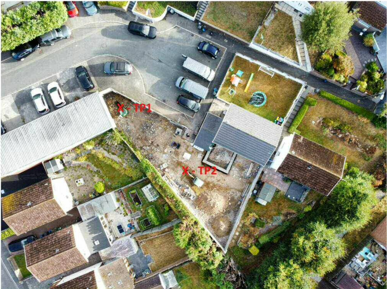
Figure 1- Test pit locations
