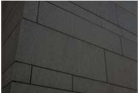
Granite Rainscreen Cladding ECC
