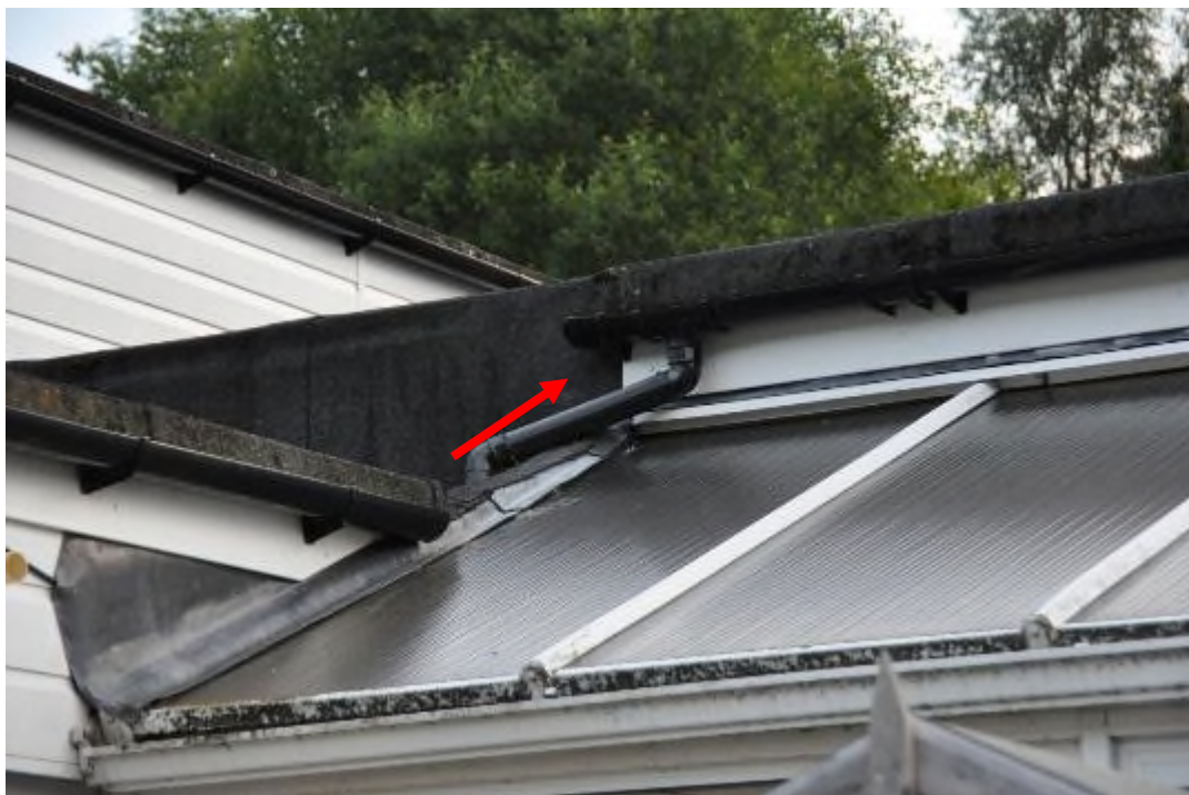
Plate 8 joints between roof areas had potential for use by bats but no evidence recorded during the survey
