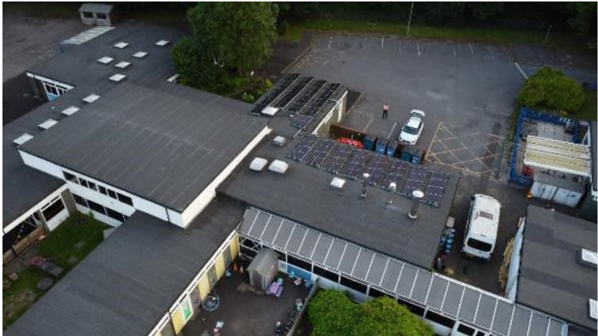
Plate 3 Roof showing no actual roof voids within the school building
