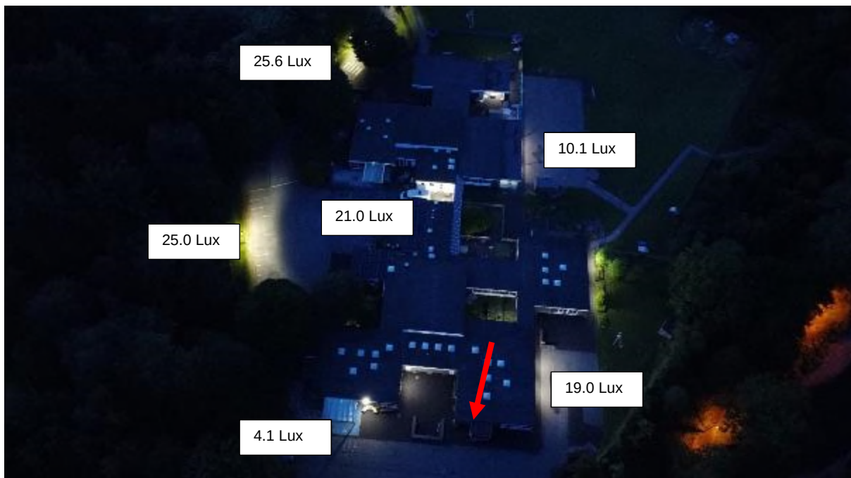
Plate 12 showing significant light spill around the property, roost arrowed
