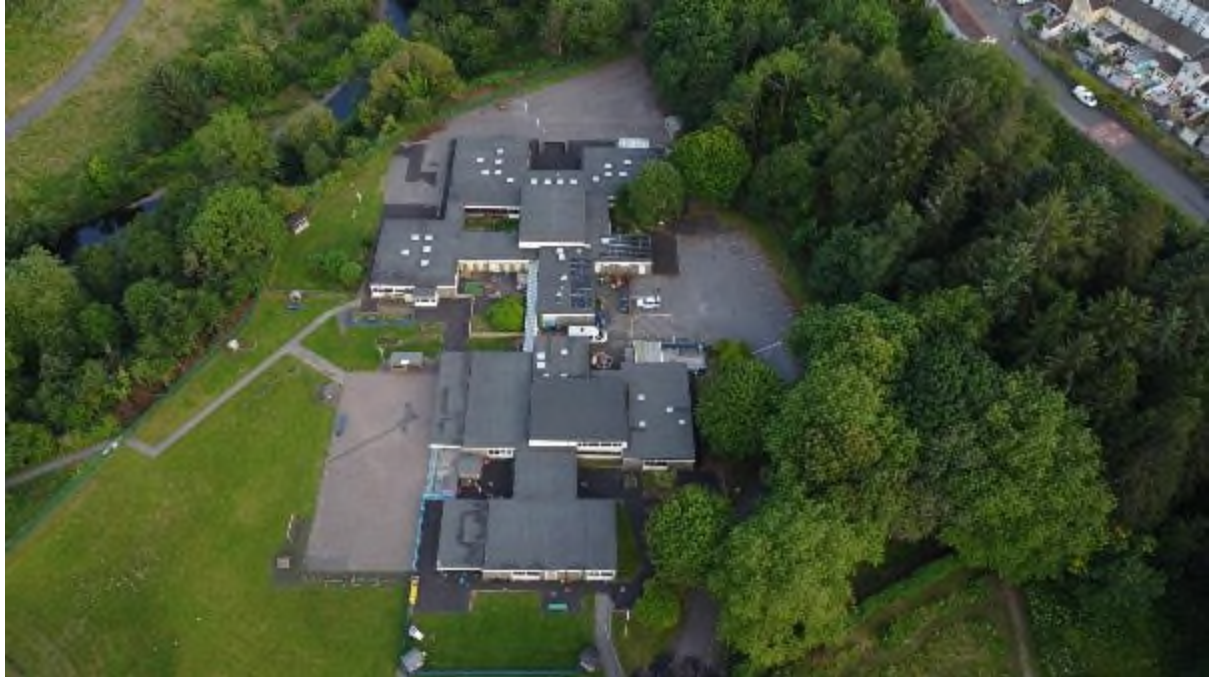
Plate 1 Building being surveyed Rhyd Y Grug School looking south
