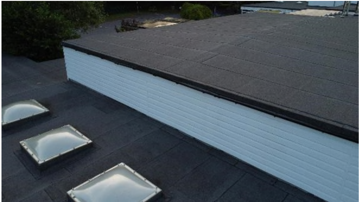
Plate 5 well maintained roof covering and weather boarding no opportunities for bats
