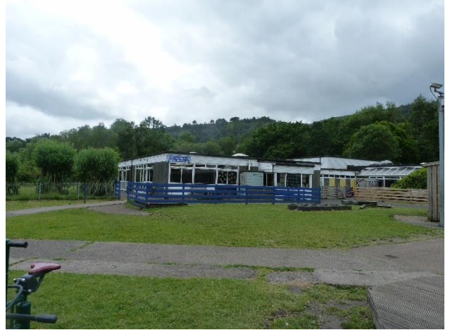
Photo 8: Eastern aspect of B1, looking south-west
