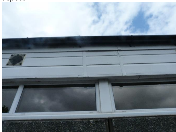
Photo 14: Gap in concrete cladding on eastern aspect leading to a crevice in cavity wall behind cladding on western aspect
