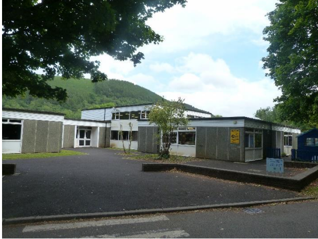
Photo 7: Western aspect of B1, looking south-east
