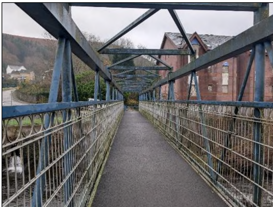
Plate 4.2 River Taff footbridge
