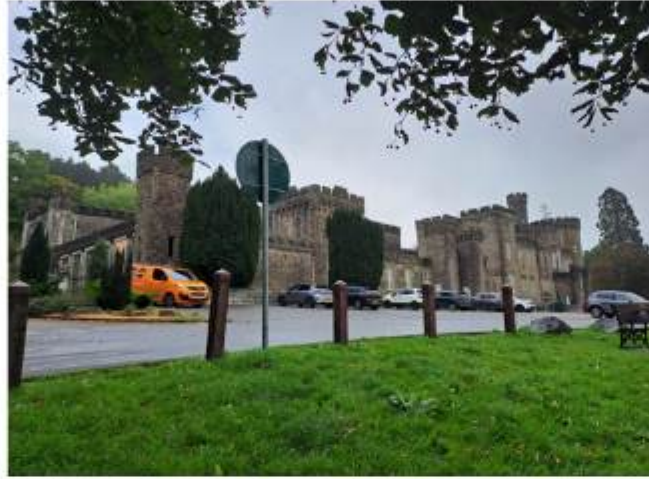
View 05. The Castle from the south-eastern approach. The south-eastern drive is marked on the 1850 Tithe Map, and has long served as a principal access route to the Castle. This constitutes a softer, less formal approach than that from the south; there are no formal gardens on this side of the Castle and the building is seen against the backdrop of the dense woodland to the north-east.
