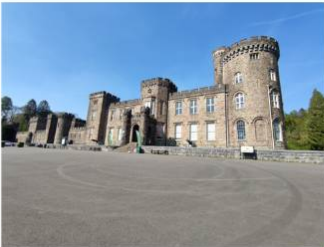
Looking across the lower terrace (car park) towards the principal elevation of the Castle.
