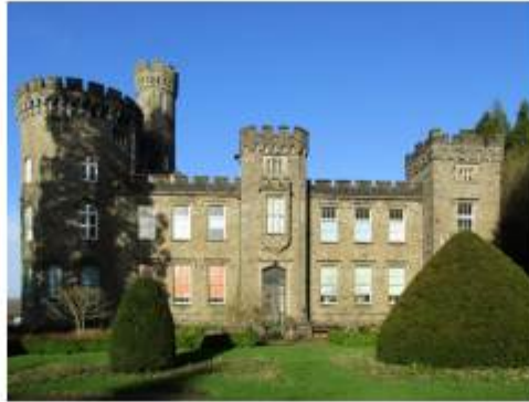
East elevation and former family entrance
