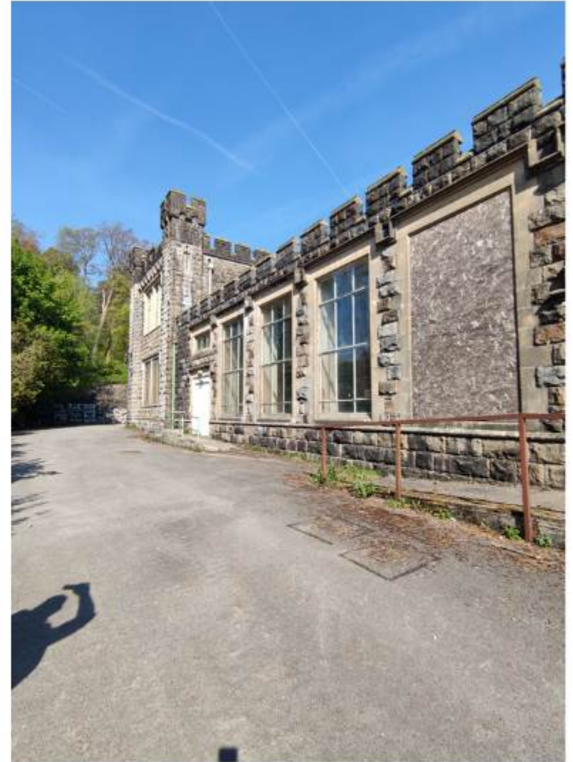
The west elevation of the Castle, showing the modern hardstanding in this area.
