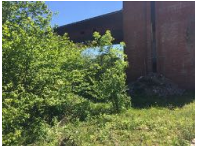
Vegetation along river at new outfall
