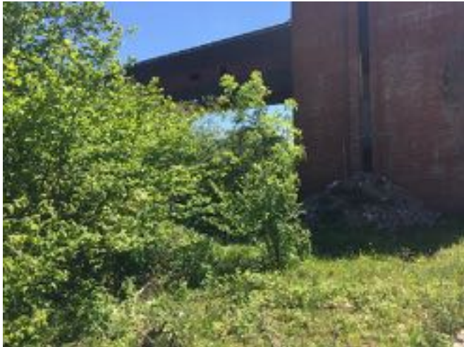
Vegetation along river at new outfall
