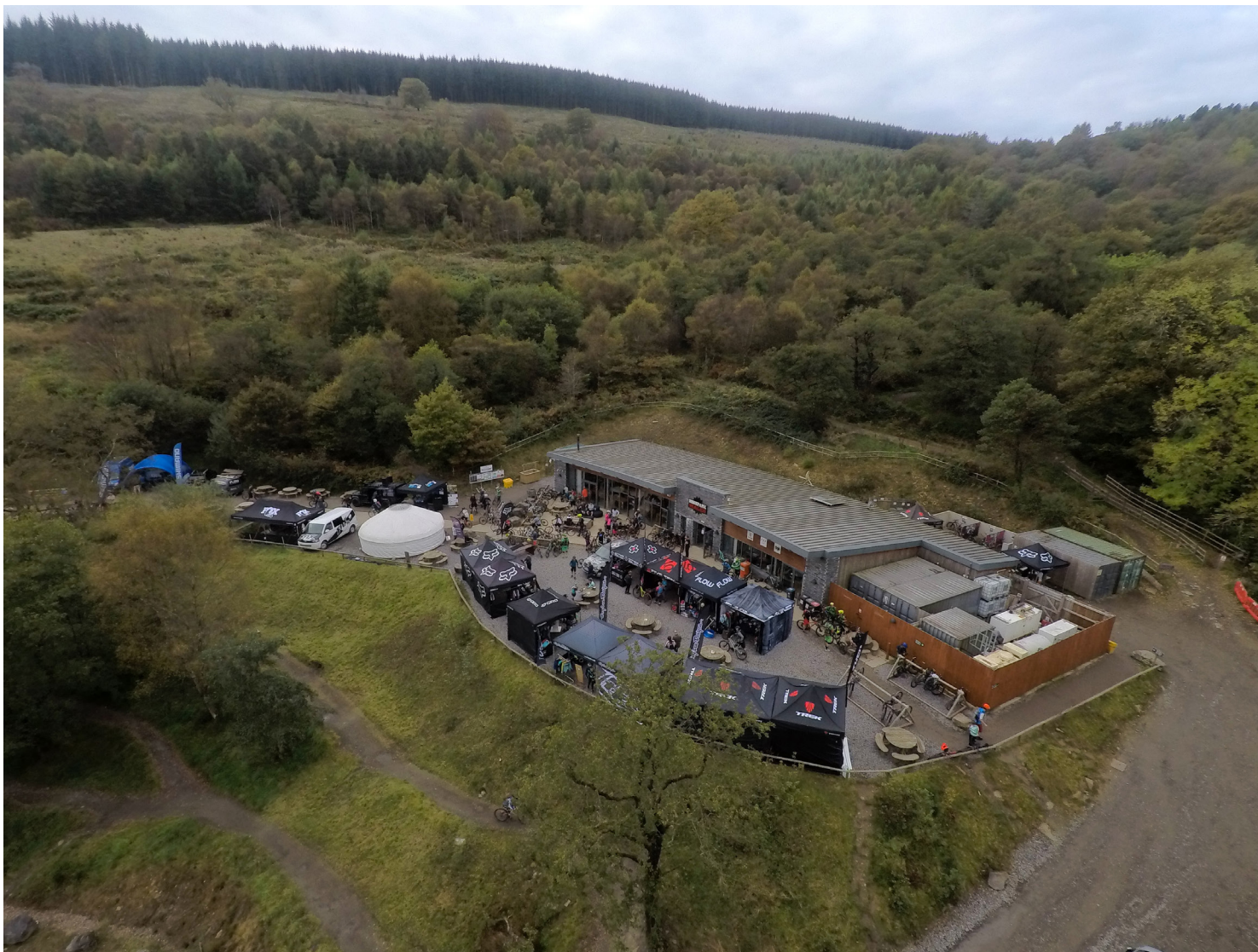
Existing BikePark Wales centre from above
