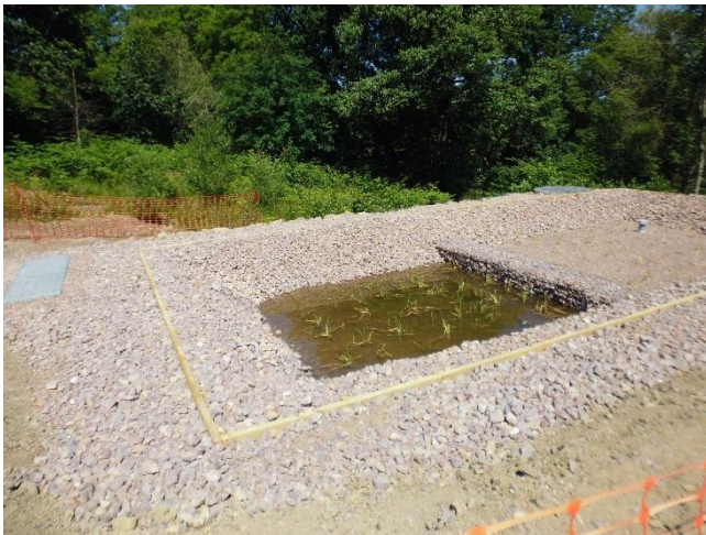
Figure 12 – Reedbed pond (new) to west of site
