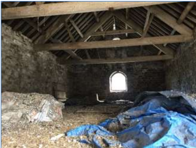
Photograph 11. Building B, western section. The first floor.
