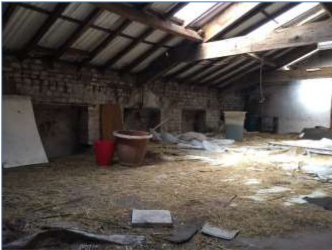
Photograph 39. Building H. The mezzanine loft level is very well lit.
