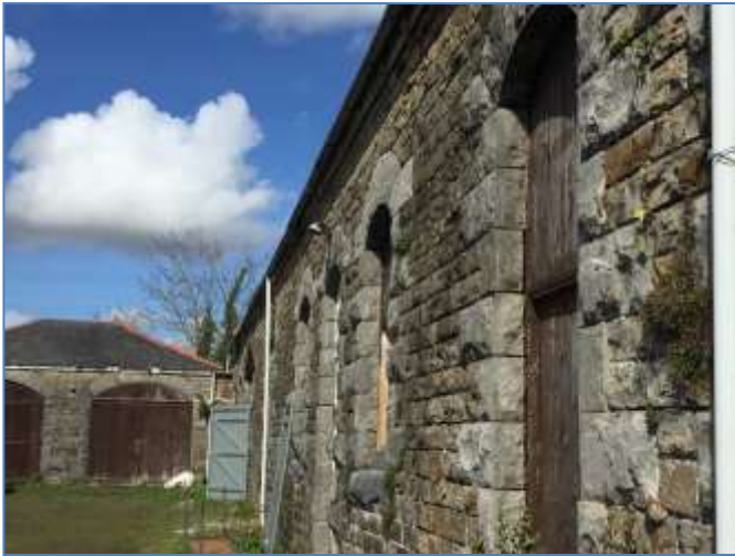
Photograph 25. Building F. The southern elevation.
