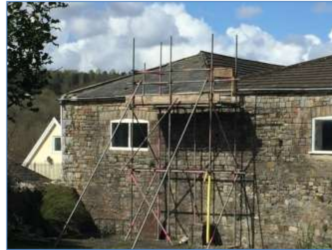
Photograph 26. Building F. The eastern elevation.
