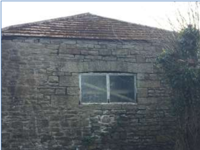
Photograph 27. Building F. The western elevation
