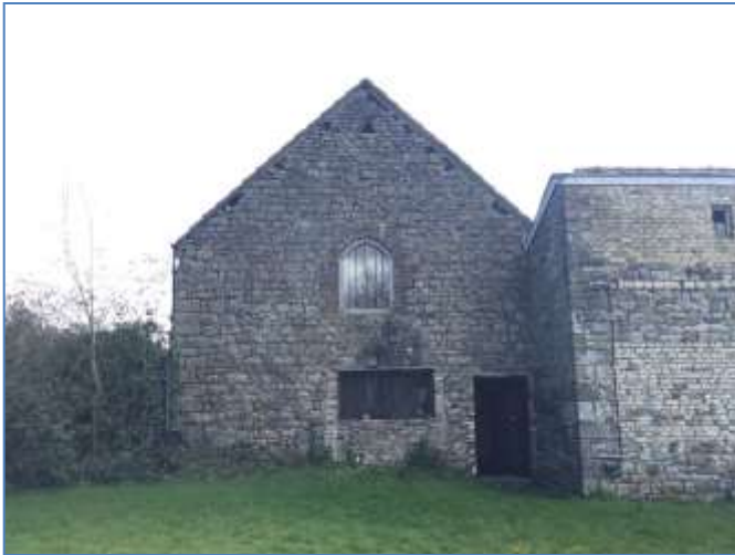
Photograph 9. Building B, western section. The western elevation (adjacent to Building C).
