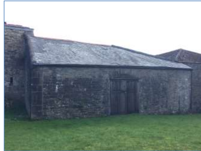
Photograph 18. Building D. The western elevation.
