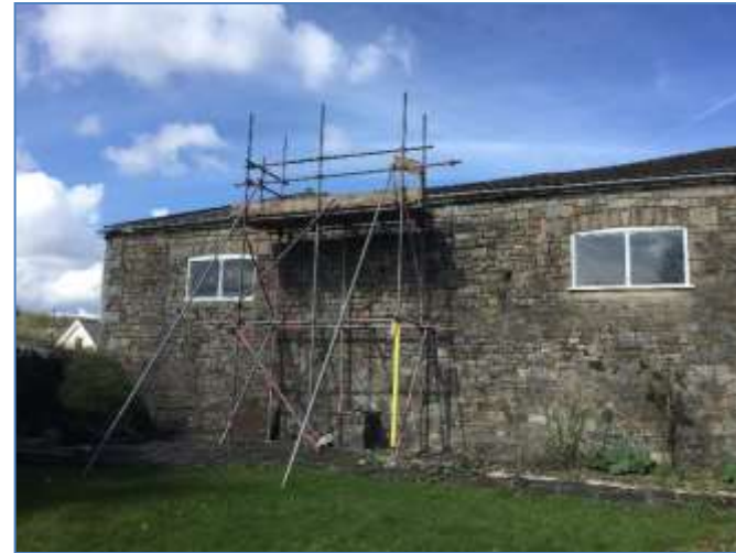
Photograph 34. Building G. The eastern elevation (right hand section of building).
