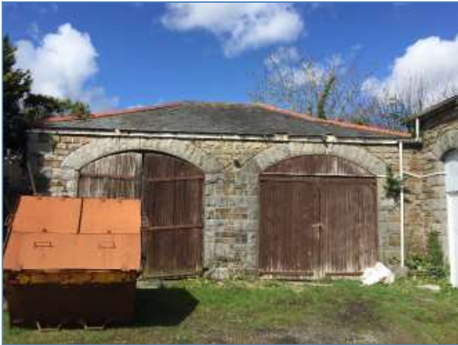
Photograph 21. Building E. The eastern elevation.
