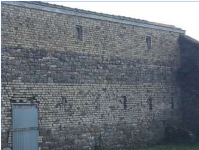
Photograph 15. Building C. The western elevation.
