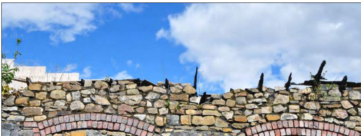
Plate 25. Remains of the burnt ceiling rafters set into the east wall
