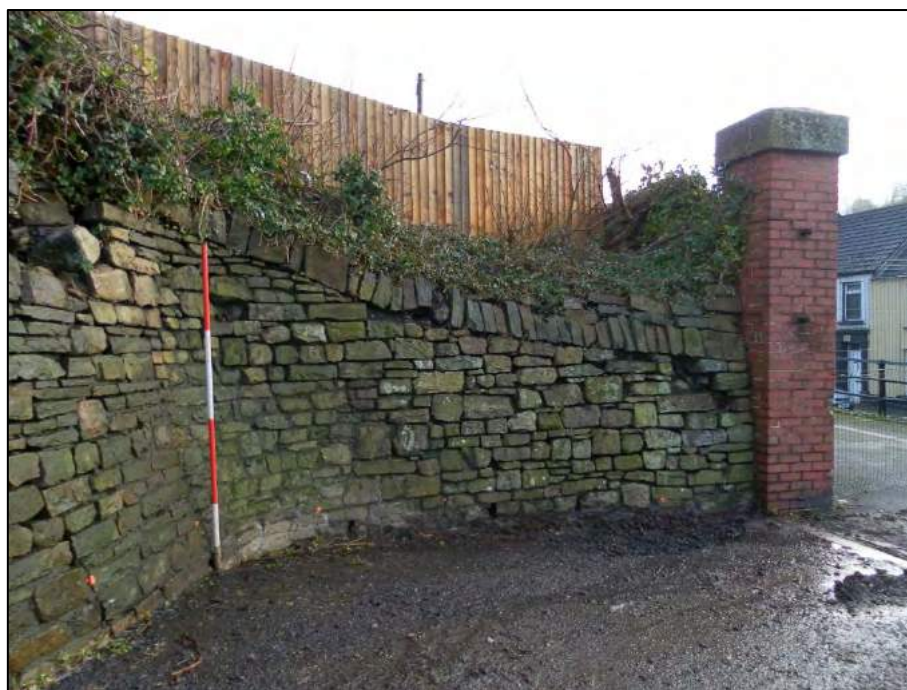
Plate 18. General view of the retaining wall 014 separating Areas D and Area A, view to south east. Scale divisions 0.5m
