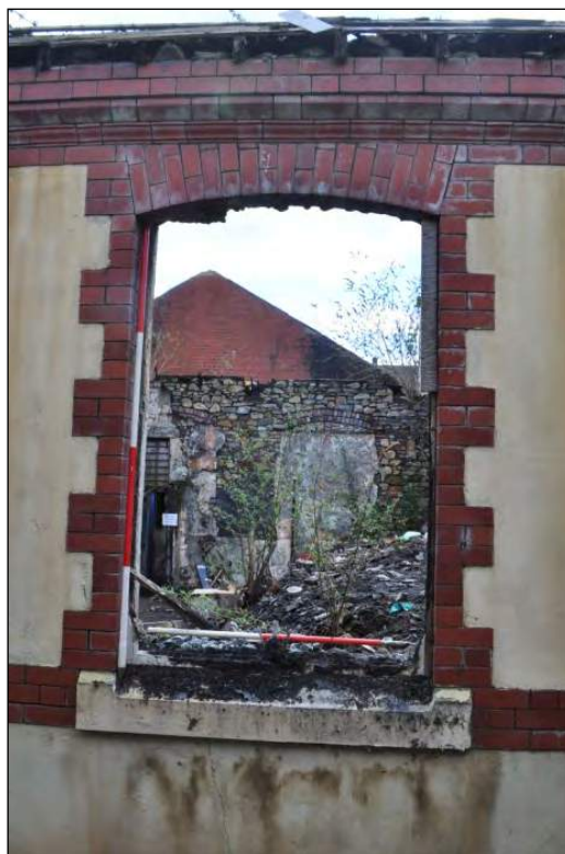
Plate 11. Close up of window exterior set into east wall of church
