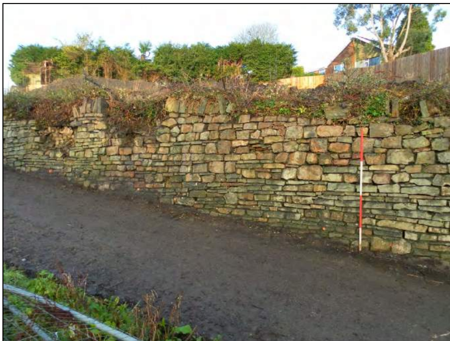
Plate 19. General view of a typical section of retaining wall 014 separating Area D and Area A showing method of laying the stone. Scale divisions 0.5m
