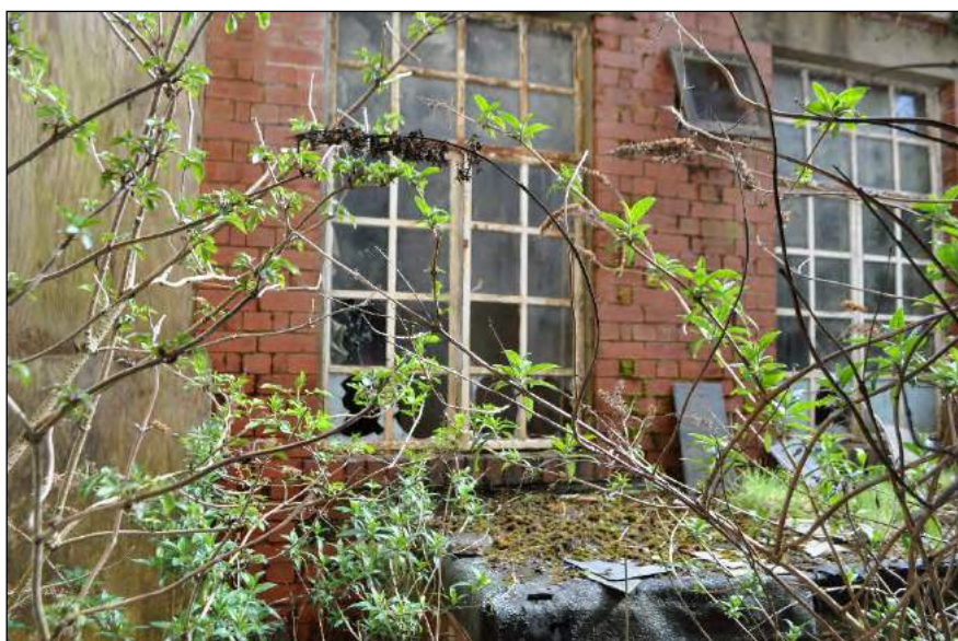
Plate 37. Rear (north side) of Labour Exchange
