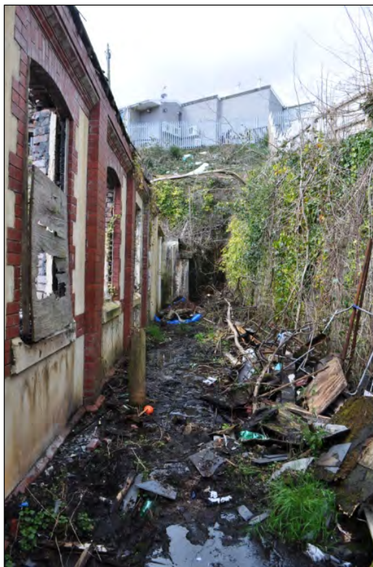
Plate 8. The exterior wall to the Labour Exchange/Chapel and perimeter retaining walls (north and east)
