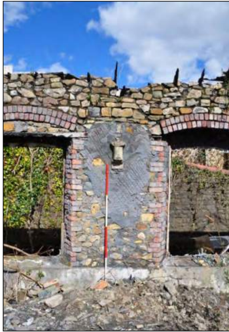
Plate 17. Internal aspect of window structure east side of church hall with Corbel bracket
