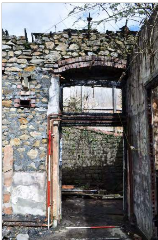
Plate 13. Close up of doorway (east side interior) in Church hall
