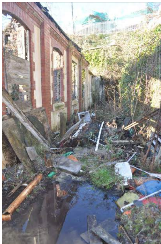
Plate 27. Showing debris and overburden associated with east side church and retaining walls
