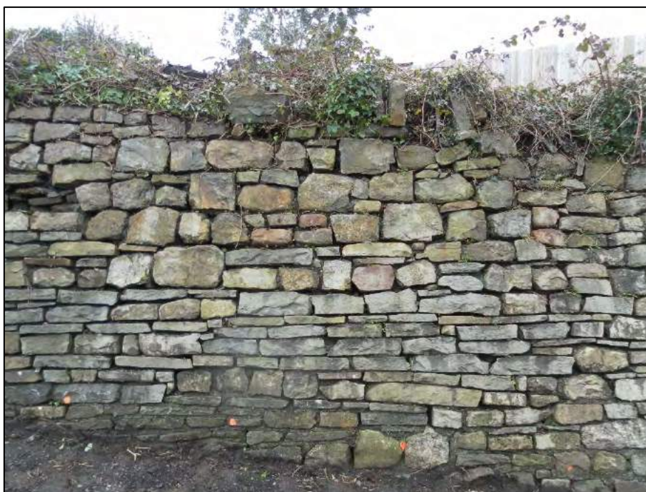
Plate 2. General photograph of the wall in the area of elevation drawing Figure 15b
