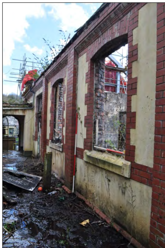
Plate 9. East wall of church looking south towards entrance
