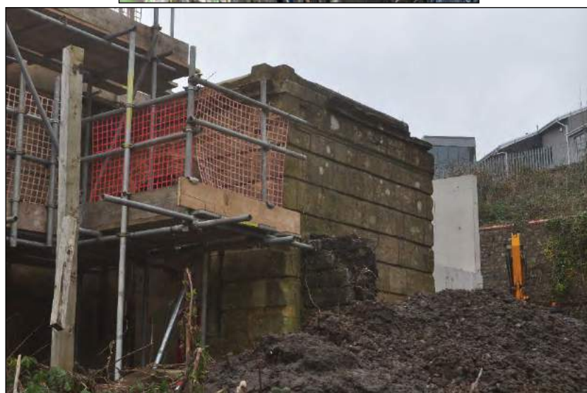
Plate 7. Detail of east entrance walling following demolition of retaining wall
