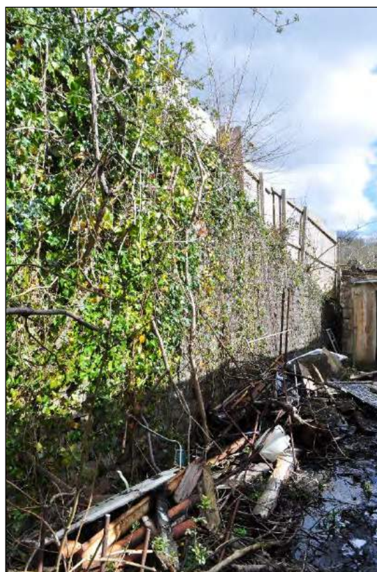
Plate 28. East side retaining wall
