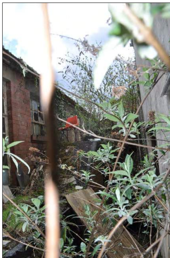
Plate 38. Rear (north side) of Labour Exchange showing level of overburden and debris
