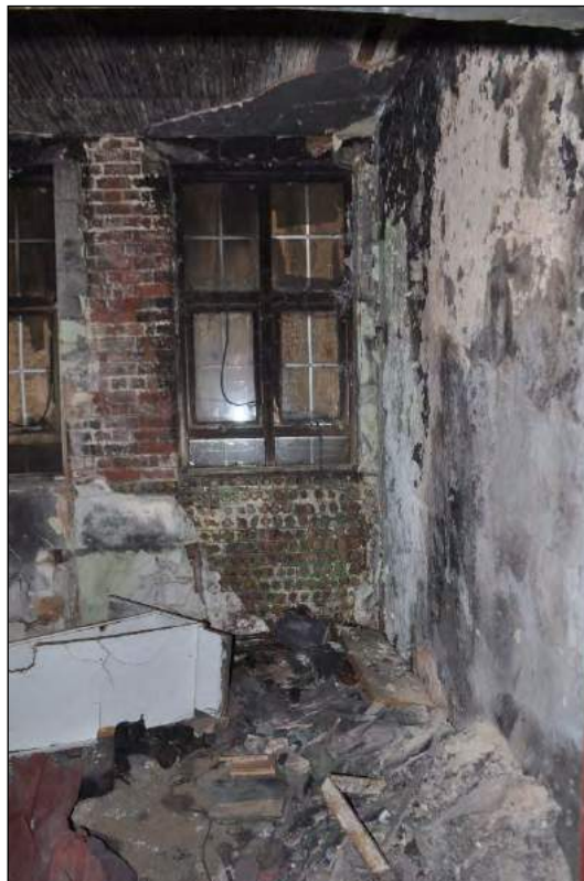
Plate 34. End room west end of Labour Exchange with lath and plaster ceiling unlike concrete panel ceiling in previous rooms
