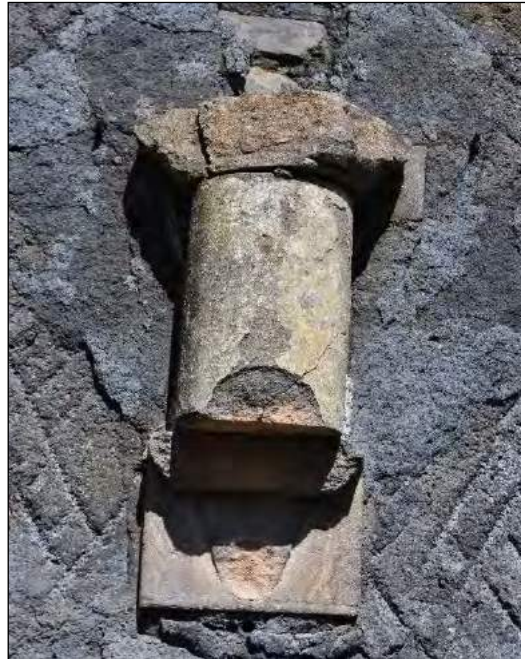
Plate 19. Detailing Corbel bracket set in east wall of the church hall
