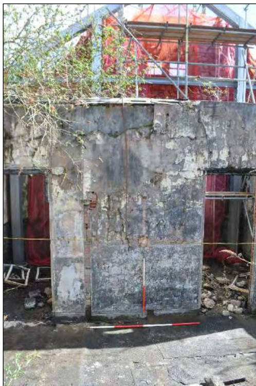
Plate 21. Rooms built into the rear of the front wall of the church looking south
