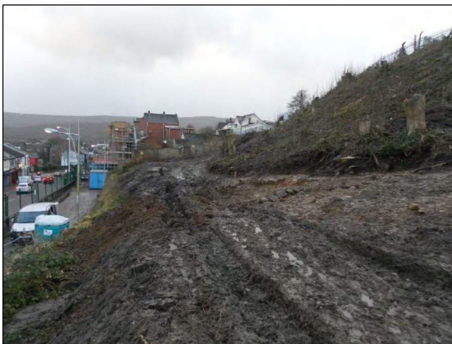
Plate 2. Development area stripped of topsoil and beginning to reveal features of interest, view to south west.
