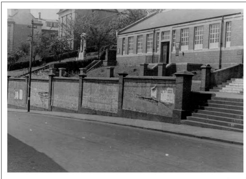
Plate 29. The Labour Exchange Building that extended and incorporated former mission church
