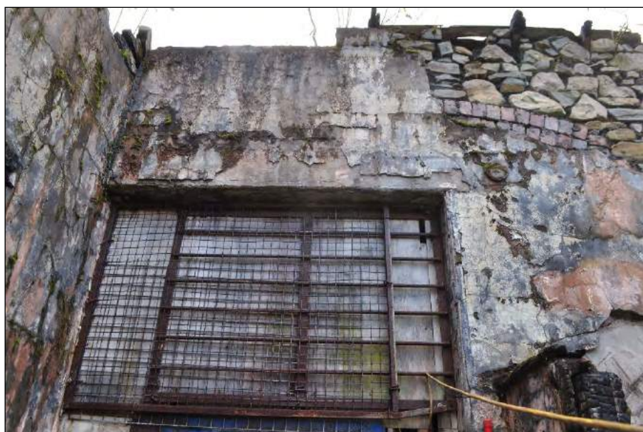
Plate 15. Window with steel grille, the brick header to the original west doorway
