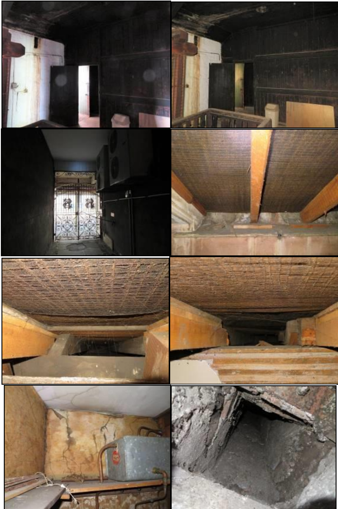
Additional interior images above the timber lining to the roof and up chimneys
