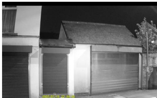
Plate A: Infrared Monitoring (NVA - Image quality)
