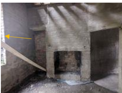
Plate 7 – Ground-floor, rear room – window opening to the courtyard.
