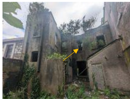
Plate 4 – Rear elevation of building B showing location of roost entrance used by greater horseshoe bat and on one occasion by a common pipistrelle.
