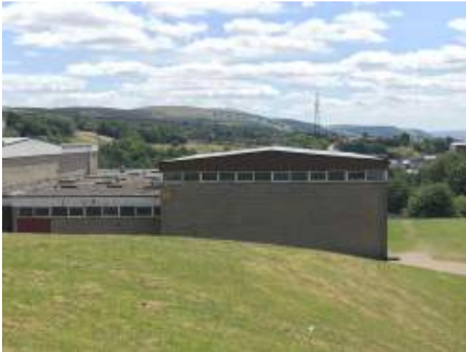
Roof view of Building 5
