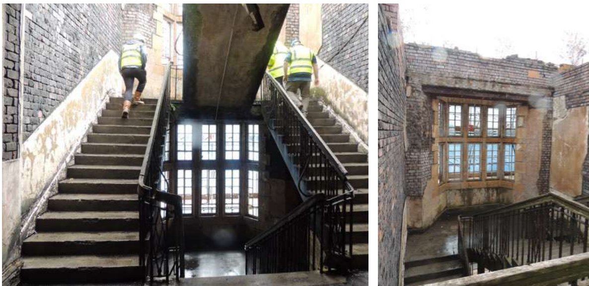
Above: The 'imperial staircase' prior to the temporary roof recently being added over. This originally provided vertical access from the ground floor main entrance to the 2nd floor.
