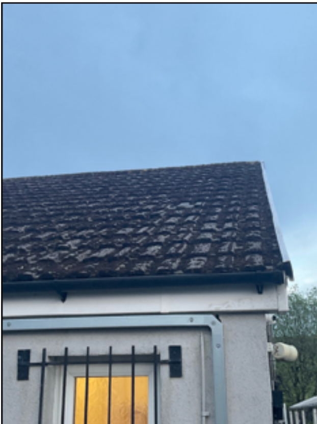
Areas of Missing Mortar Between Tiles
