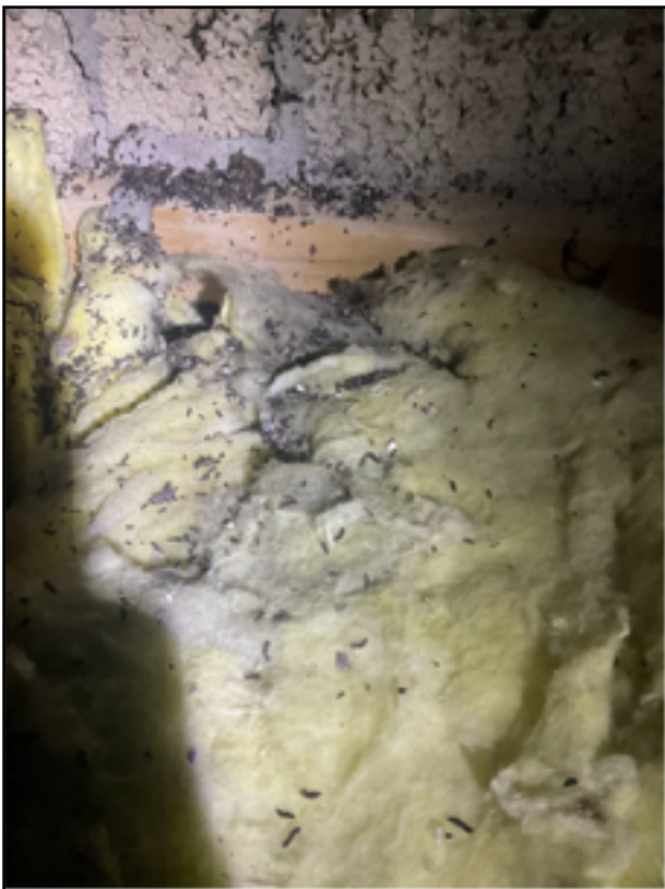
Accumulation of Bat Droppings (NW End)
