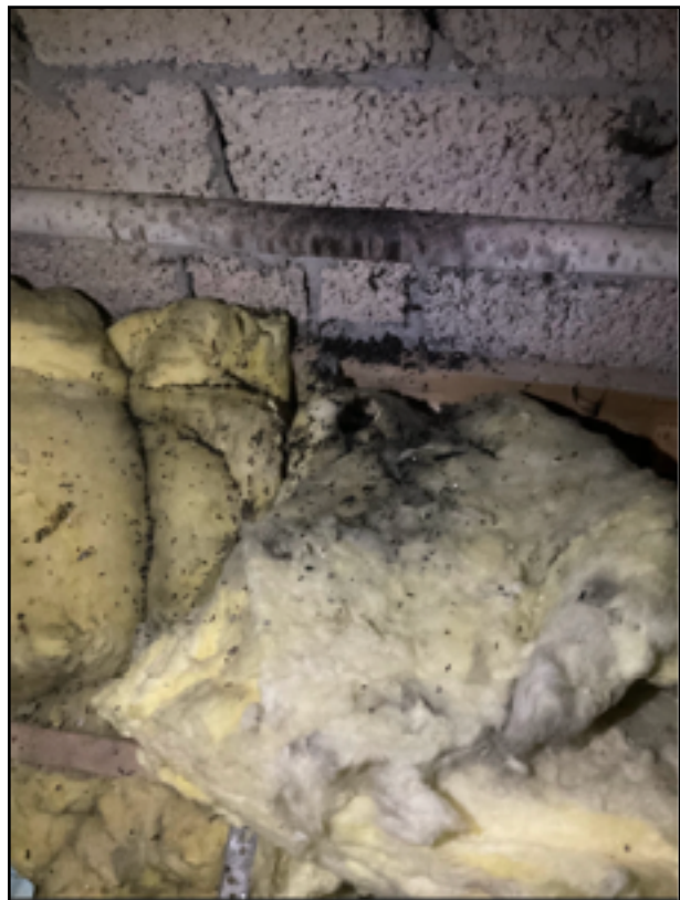
Accumulation of Bat Droppings (NW End)
