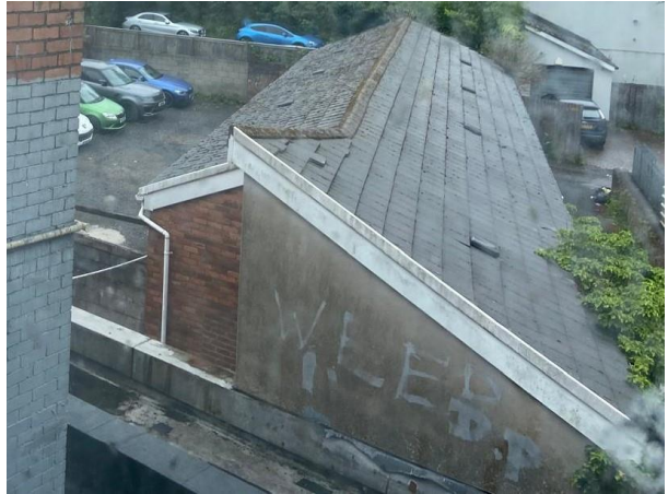
Photo 17: Western Elevation and View of the Roof
