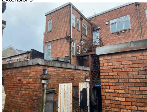
Photo 2: Eastern Rear Showing Single-storey Extensions
