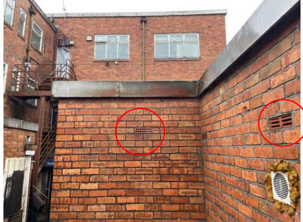
Photo 8: Example of Vents on the Single-storey Extensions
