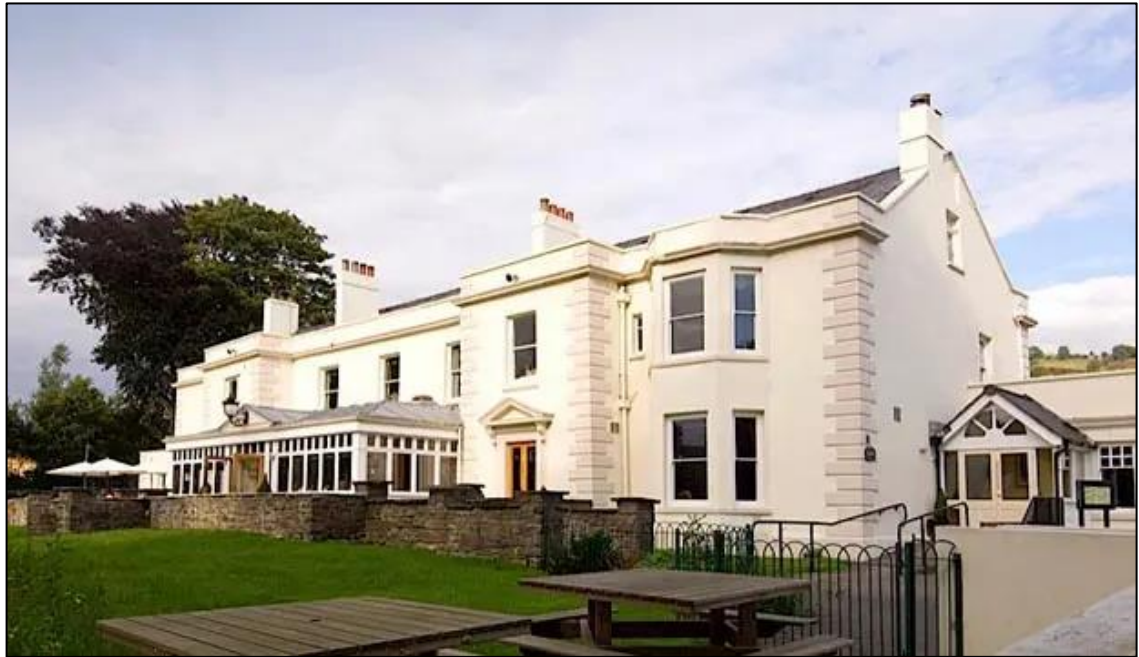
Figure 1 Premier Inn Merthyr Tydfil (Source. Premier Inn (2025))
