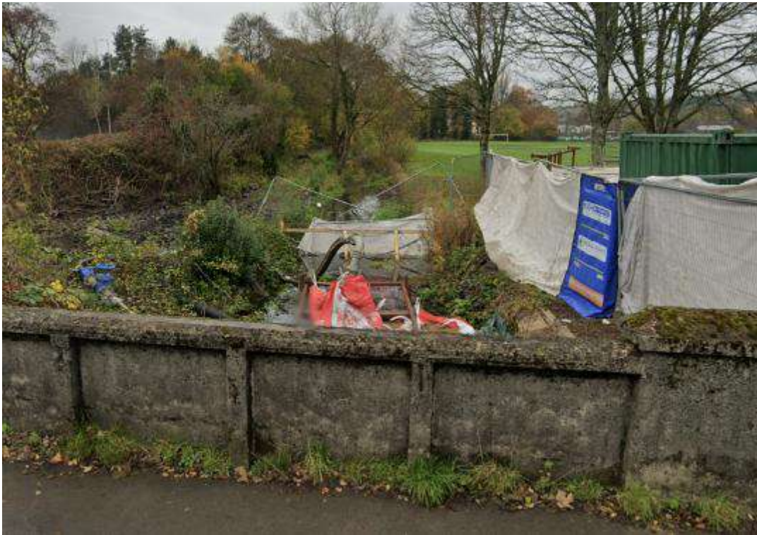
Figure 8: View of improvement works at Maestaff Street Bridge (looking north west)
