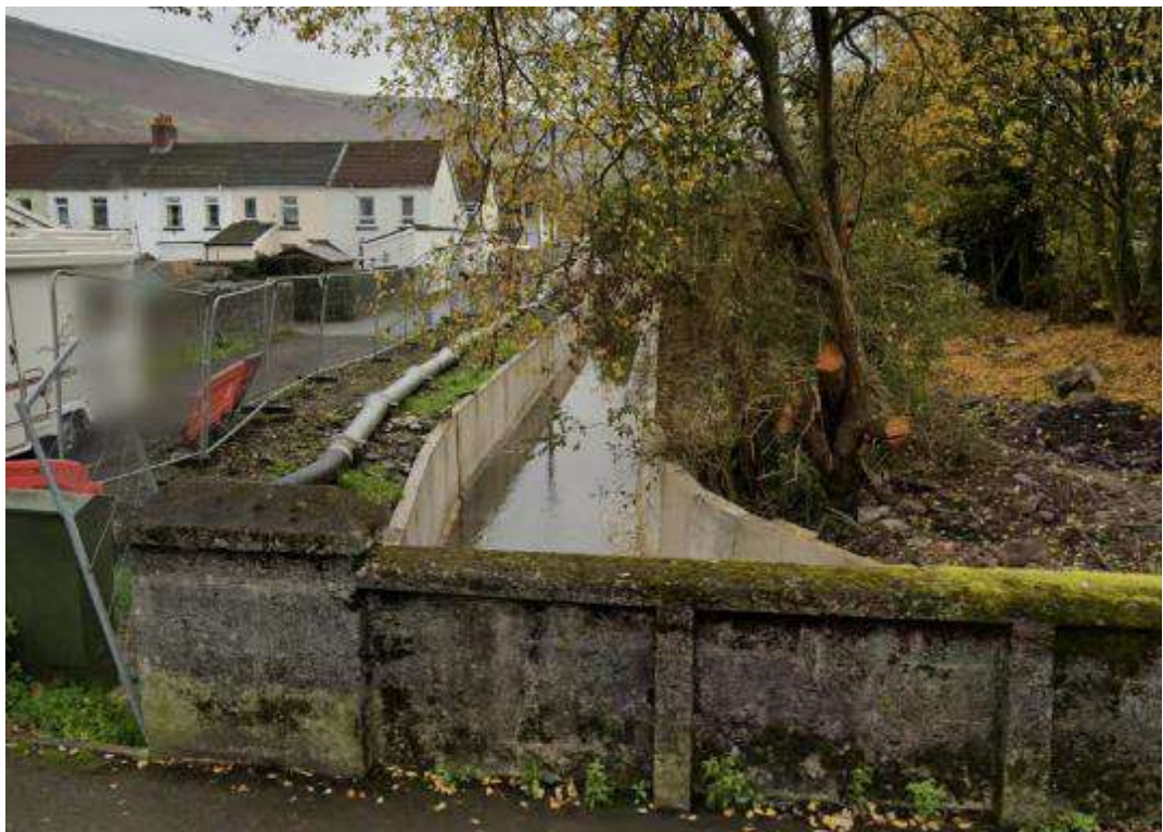
Figure 9: View of improvement works at Maestaff Street Bridge (looking south east)
