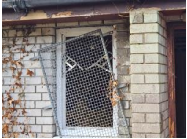
Photo 16: Broken Glass Panels in Door
