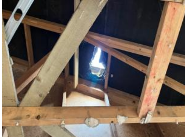
Photo 18: Tear in Bitumen Felt Roof Lining
