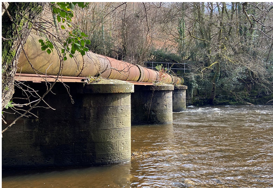
Figure 1-2: Existing Bridge Structure
