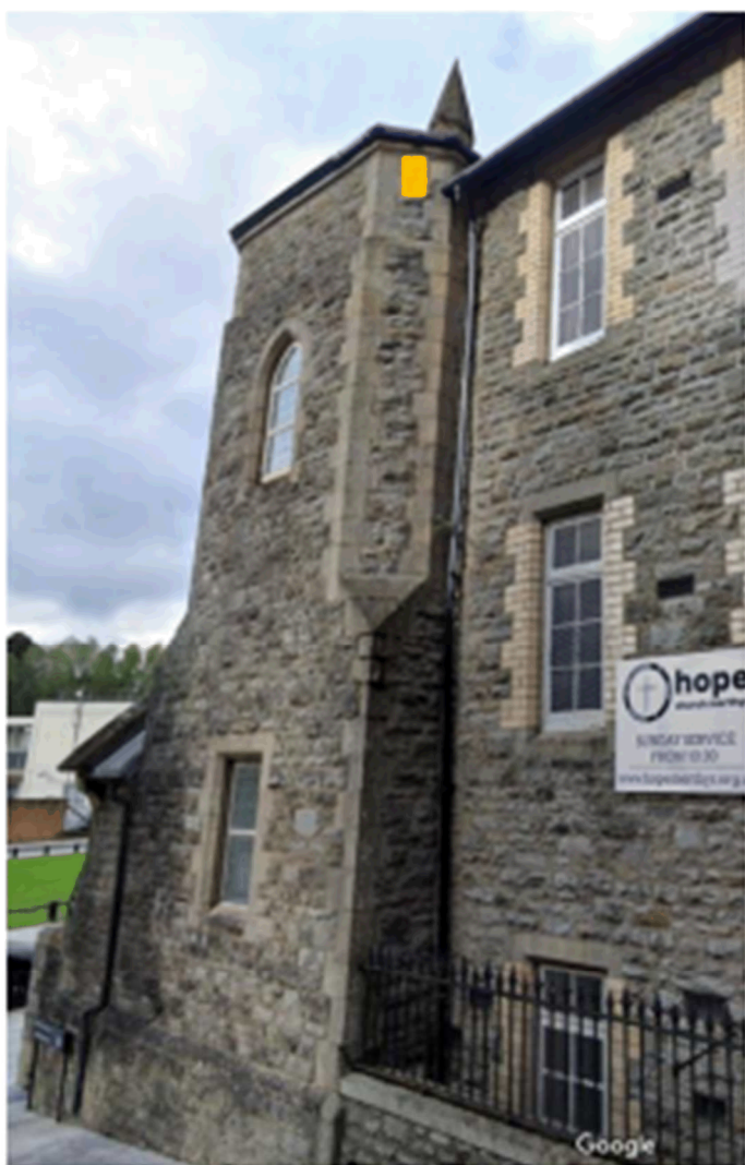
Figure 2: orange box = bat box example. Two boxes, one on either side of the building.
