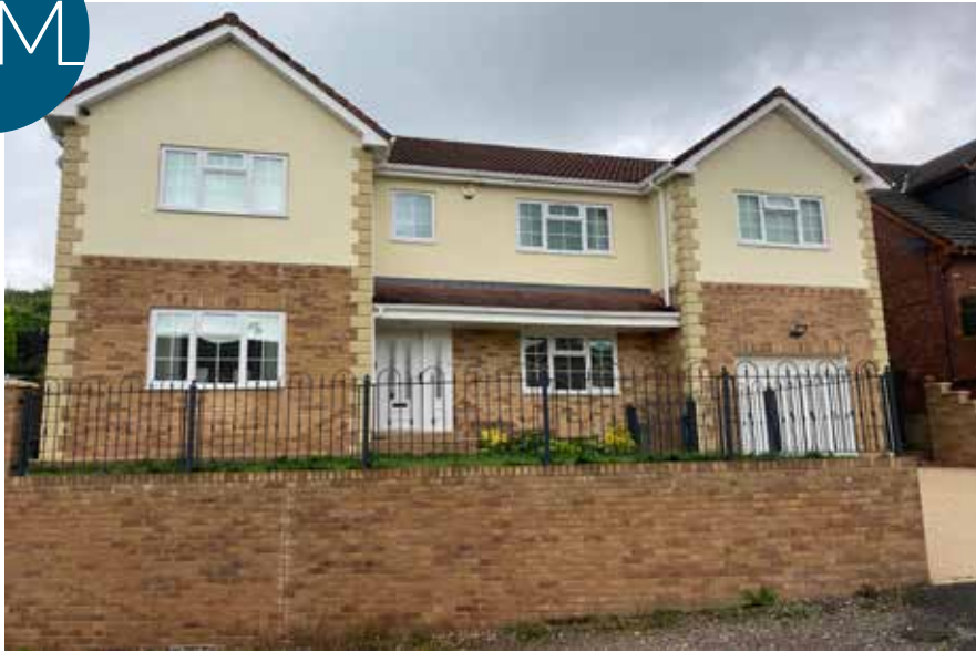
Figure 13 - Dwellings of Springfield Rise east of the site
