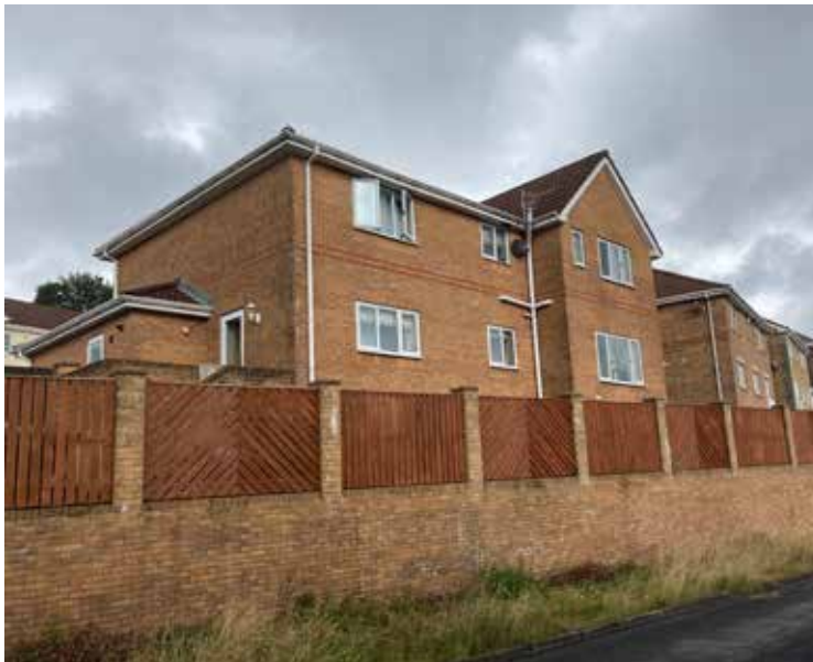
Figure 10 - Dwellings of Springfield Rise east of the site
