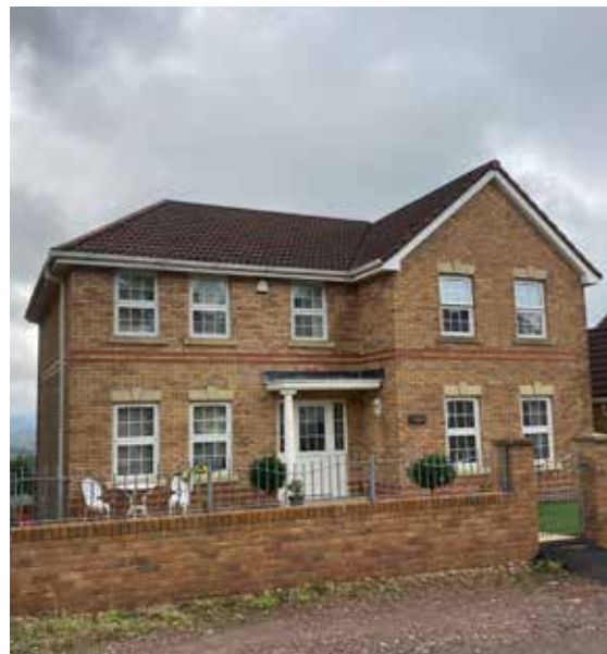
Figure 16 - Dwellings of Springfield Rise east of the site
