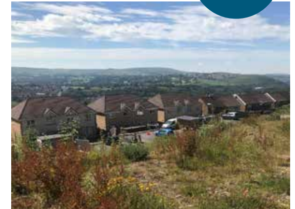
Rear gardens comprise of parking spaces/ car ports and steps to usable garden area.
