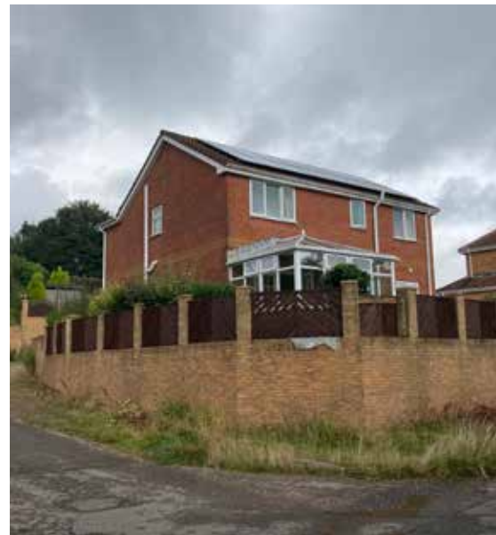
Figure 11 - Dwellings of Springfield Rise east of the site
