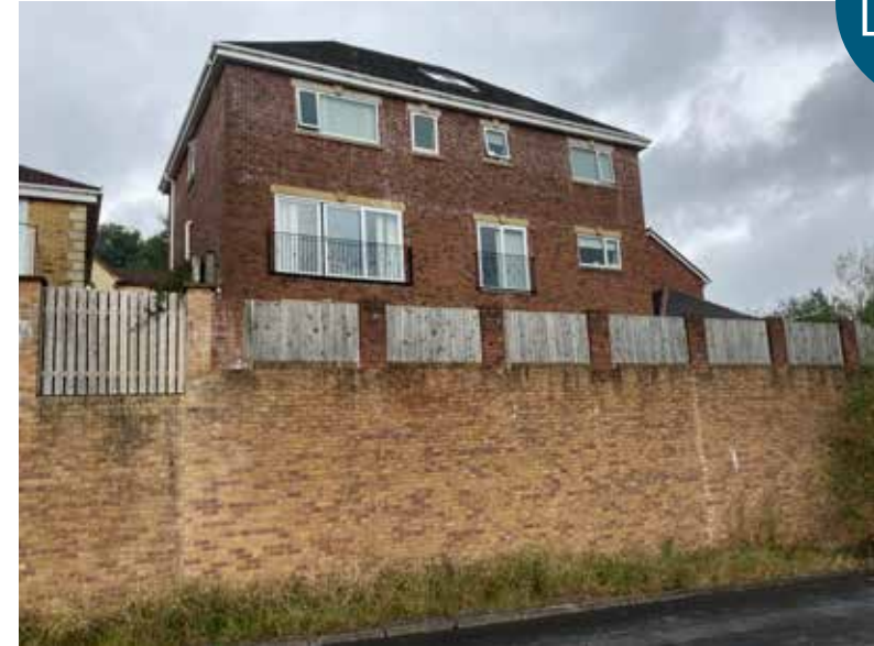
Figure 9 - Dwellings of Springfield Rise east of the site
