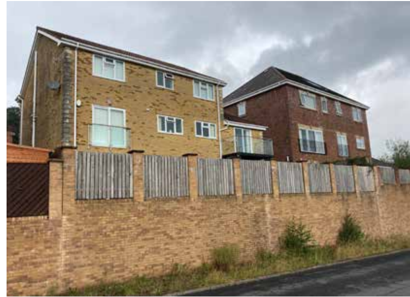
Figure 14 - Dwellings of Springfield Rise east of the site
