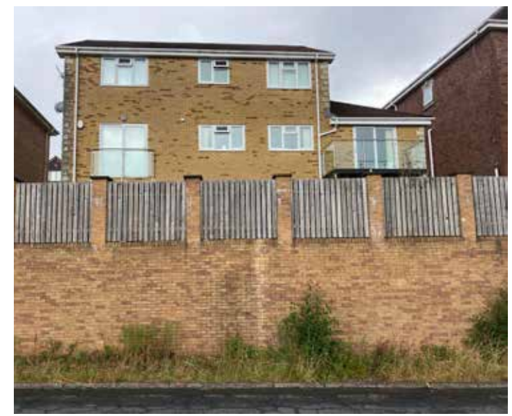
Figure 12 - Dwellings of Springfield Rise east of the site
