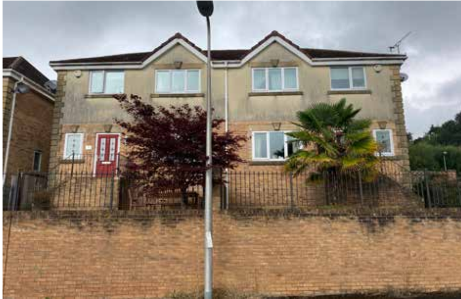
Figure 8 - Semi-detached dwellings of Springfield Rise south-east of the site
