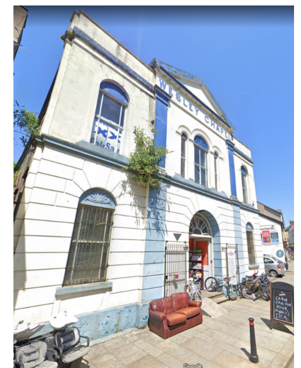
Former Wesley Methodist Church
